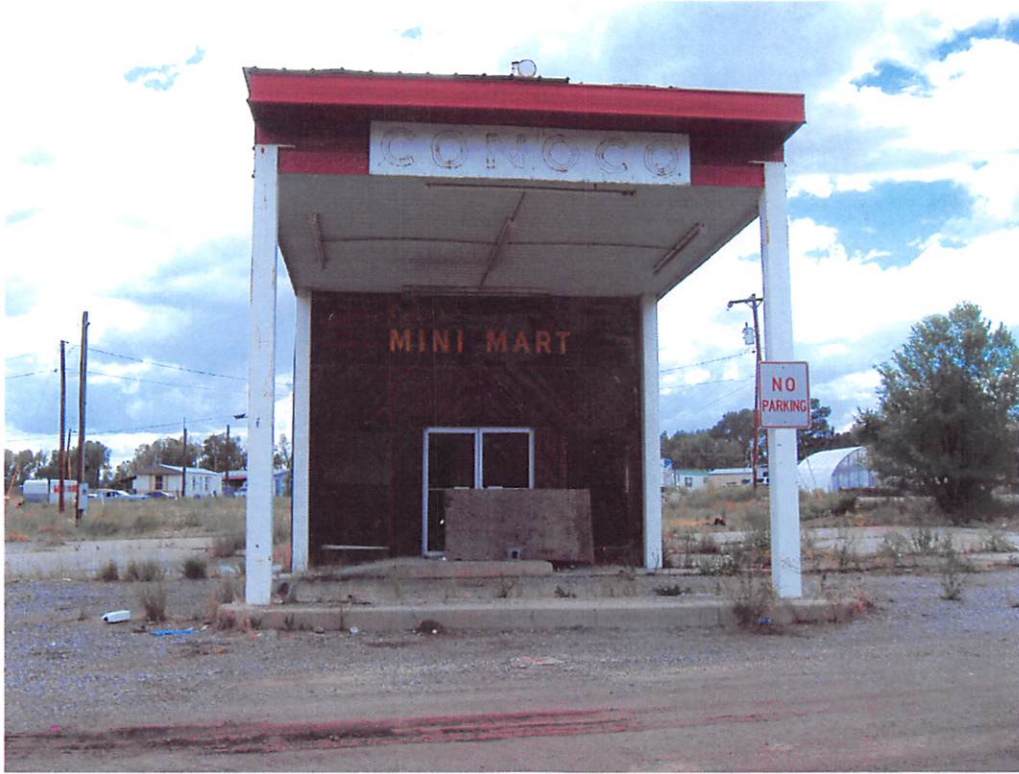
Photo 1: View of former pump islands and east side of building.
