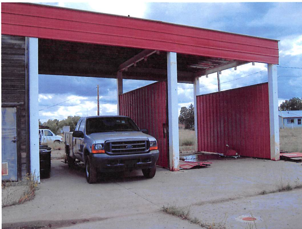
Photo 4: Car wash bays on west side of property.
