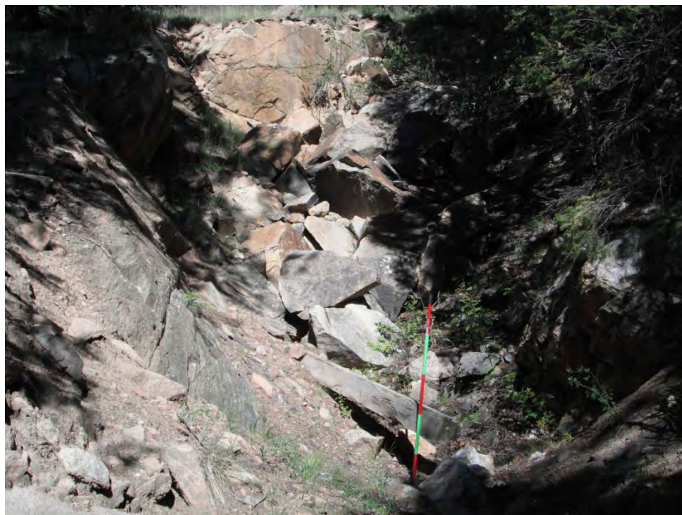
Photo 2-Looking north at Trench-1.
