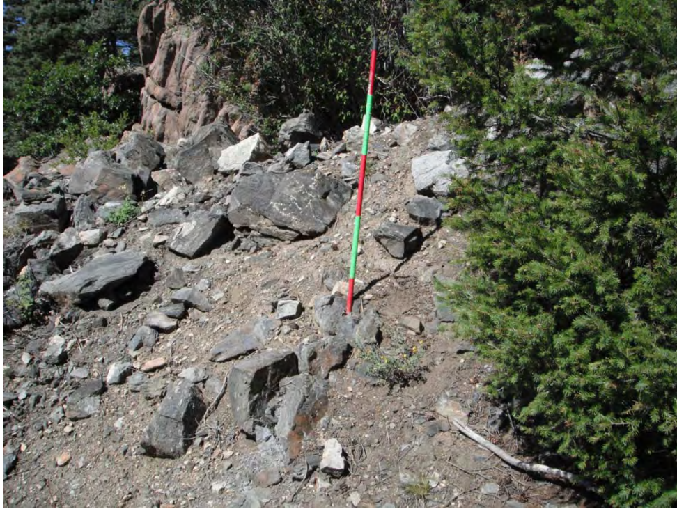
Photo 5-Looking west at PilePly-1.
