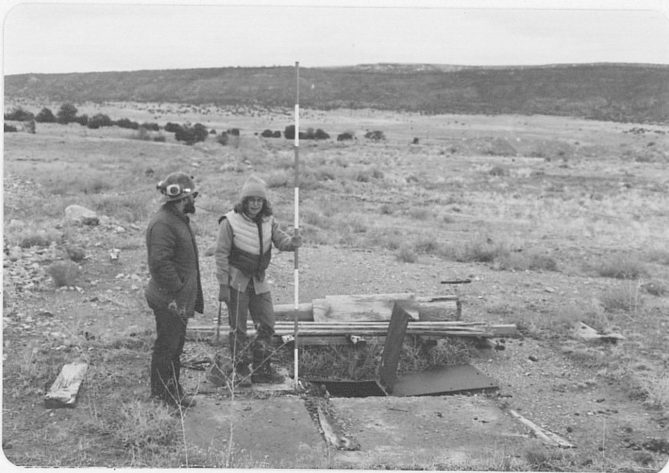
Photo (a) Close-up of T-20 shaft opening, showing concrete slab with rectangular opening covered with plate metal door.
