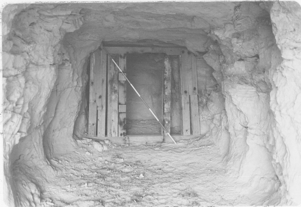
Photo (f) Partition 30' inside northernmost adit.
