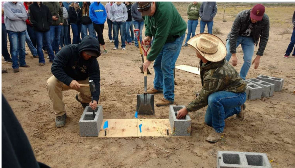
Figure 10. STEM Partnership interns took the lead in construction of sediment traps (Jeremy Gillette (left) and Dillon Hancock (right)). The base is plyboard anchored by rebar pegs. Three sides are built around the plyboard out of anchored cinder blocks.
