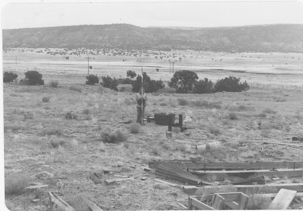
Photo D Looking east at hoisting shaft site, 1000' south of main shaft; a raised cylindrical metal lined vent protrudes about 1' above the concrete cover on shaft (arrow).
