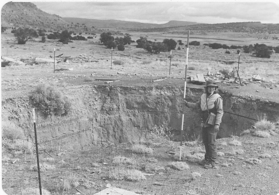
Photo B Look NE at caved shaft; enclosing fence is effective for livestock, not for people.
