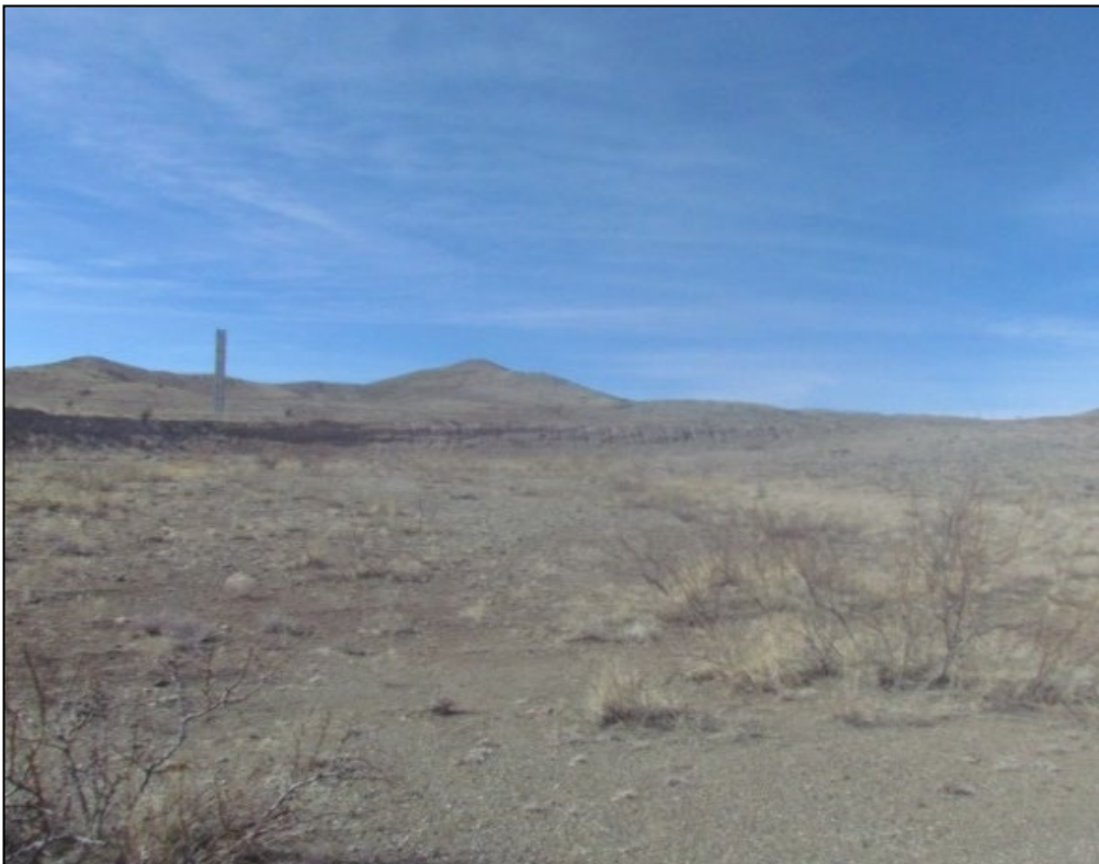
Figure 3-30. View of Tailing Pond and Tower
