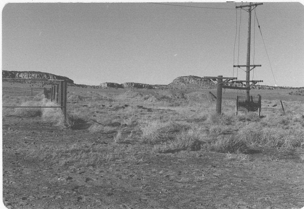
Photo (d) View northward at east fence line of the mine shaft; note small dump at center and right and electric utility line.
