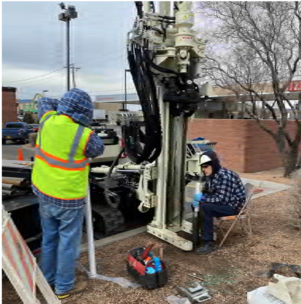
Photo 4 – Constructing well in MW-24 bore hole.
