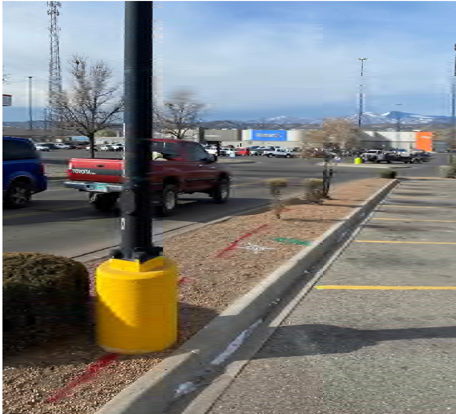
Photo 1 – Planned MW-25 location with conflicting underground electric utility locate
