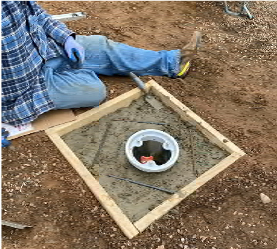
Photo 5 – Constructing wellhead at MW-24.
