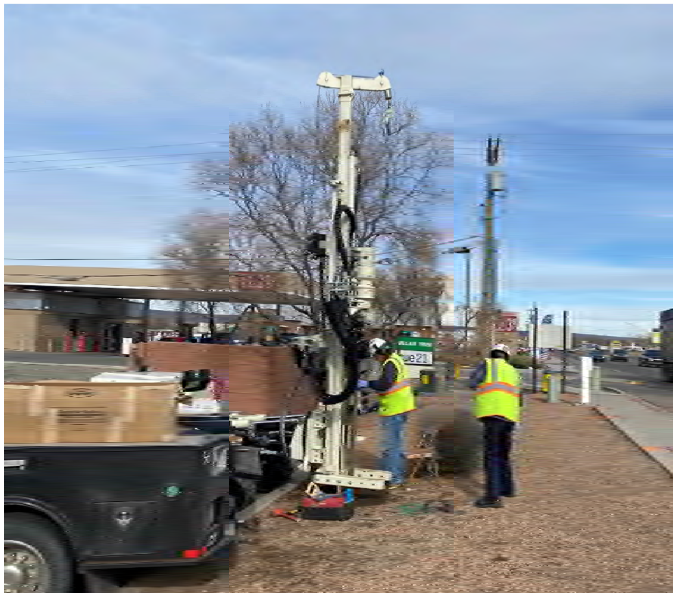
Photo 2 – Geoprobe drill rig soil sampling at MW-24
