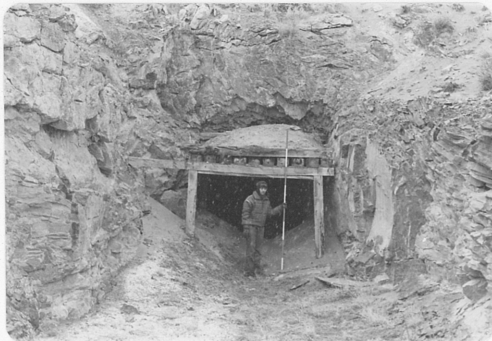
Photo (j) Close up of adit shown in (i); portal is 6' high, 7' wide, and timbered in about 20'.
