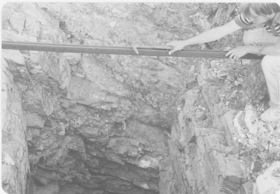
Photo (i) Vertical shaft, 6' x 6', at least 50' deep, in E \frac{1}{2} SW \frac{1}{4} , sec. 25.
