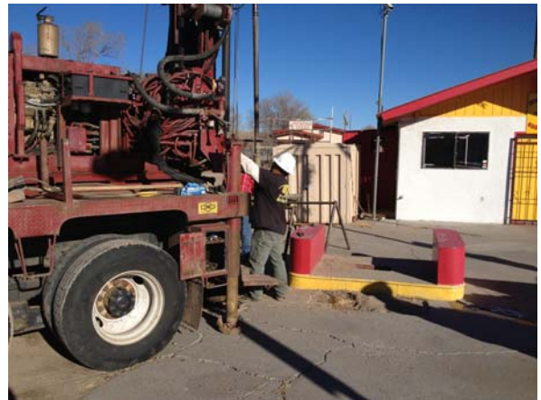
Photo #2 Advancement of soil boring B-2.
