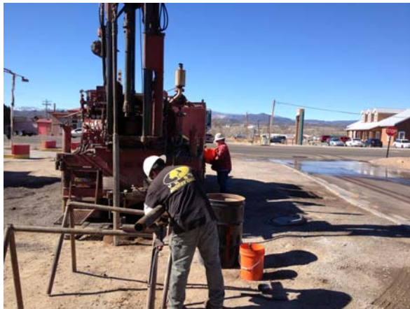
Photo #1 Advancement of soil boring B-1.
