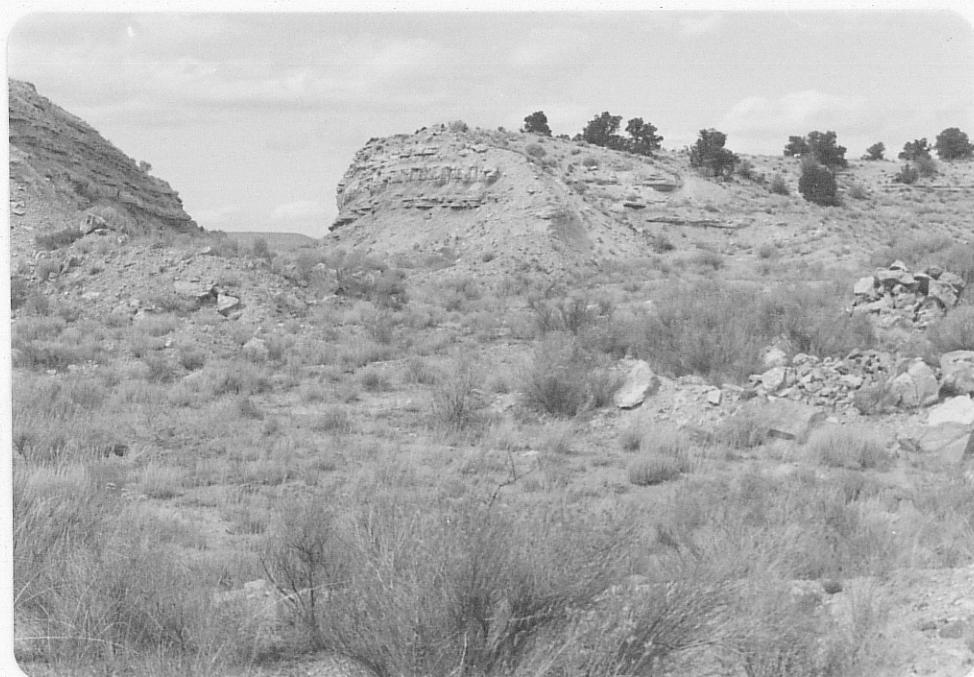
Photo (a) Looking northwest into Box Canyon Mine; cut is generally 35' wide (wider at east end), and 260' long. Small waste piles in foreground produced scintillometer readings up to 1,200 cps.
