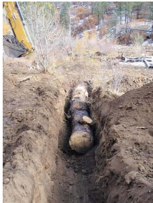
2009 – Rangeland Hands, Inc. Installing Log Vane
