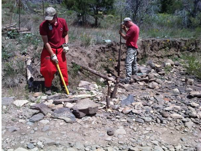
2011 – Philmont Conservation Crew installing post vanes Low-Water Crossing #3
