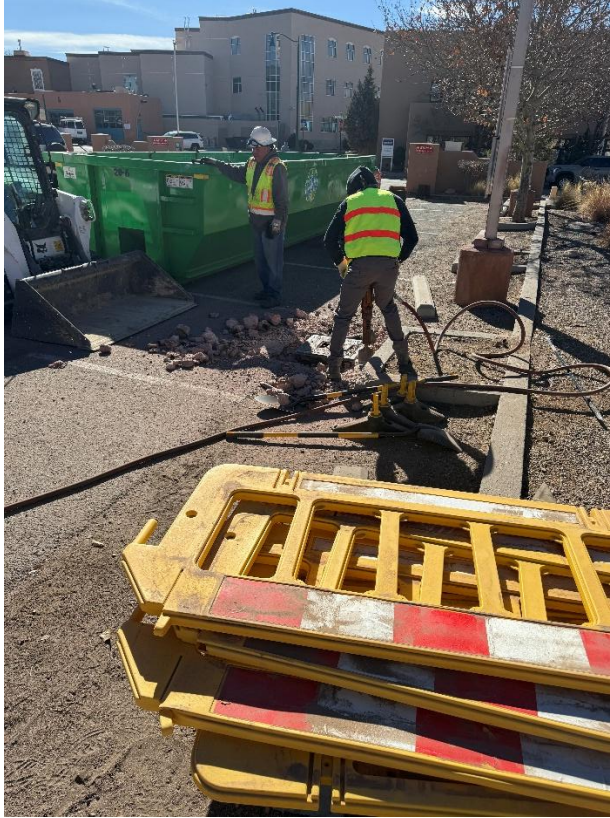
Photograph No. 5 Description: Removing the AI-2 concrete pad.
