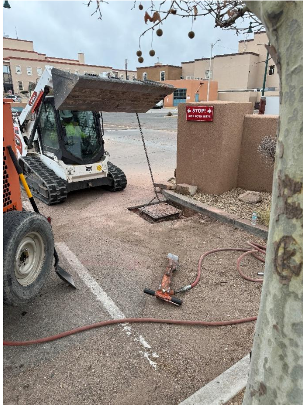
Photograph No. 9 Description: Removing the AI-1 well vault.
