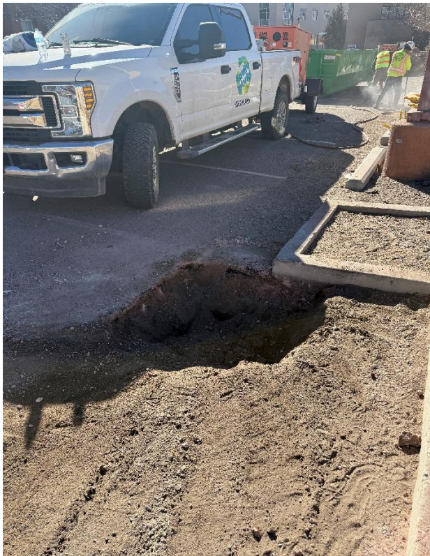
Photograph No. 4 Description: SVE-7 well vault removed.
