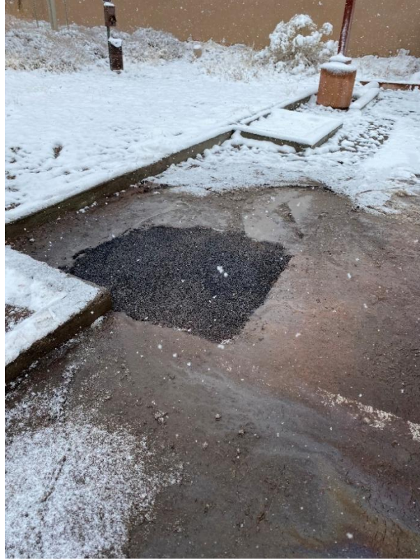
Photograph No. 11 Description: SVE-7 well vault removed and surface repair completed.
