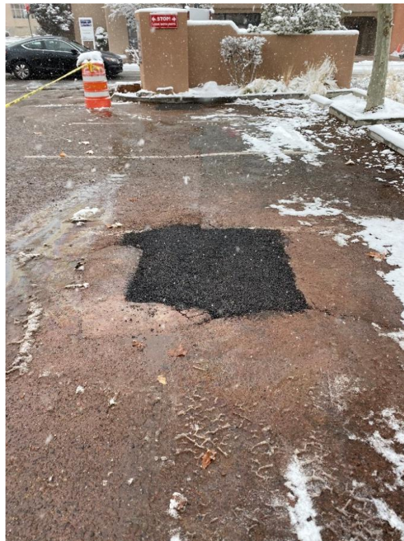
Photograph No. 12 Description: SVE-6 well vault removed and surface repair completed.
