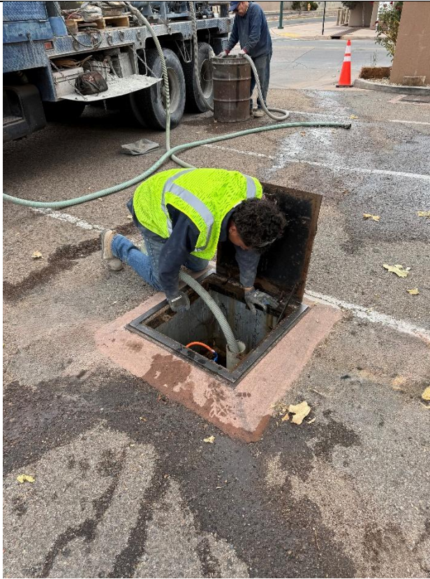
Photograph No. 3 Description: Grouting well SVE-6.
