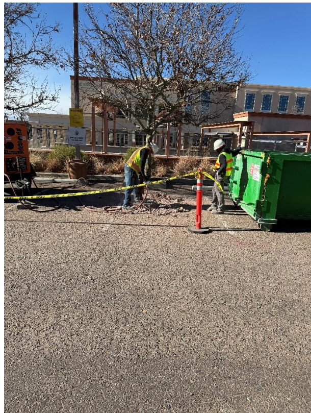
Photograph No. 6 Description: Removing the SVE-6 concrete pad.
