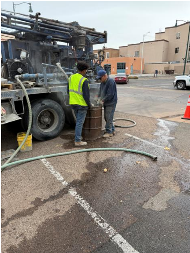
Photograph No. 2 Description: Mixing grout for well P&A.
