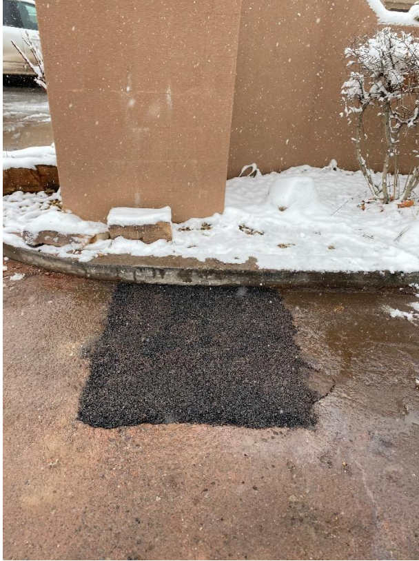
Photograph No. 13 Description: AI-1 well vault removed and surface repair completed.
