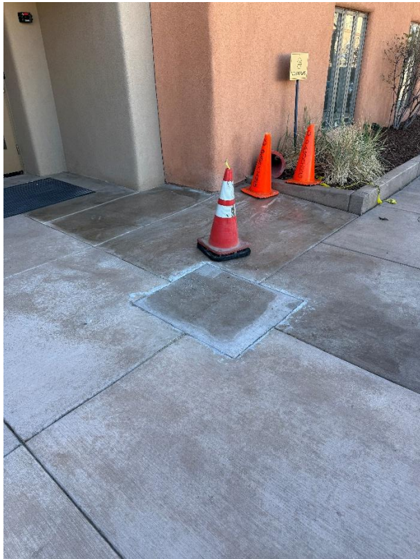
Photograph No. 14 Description: SVE-2 well vault removed and surface repair completed.
