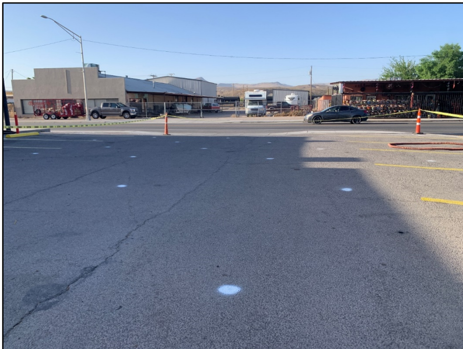
Photo 2. Pre-marked injection locations.
