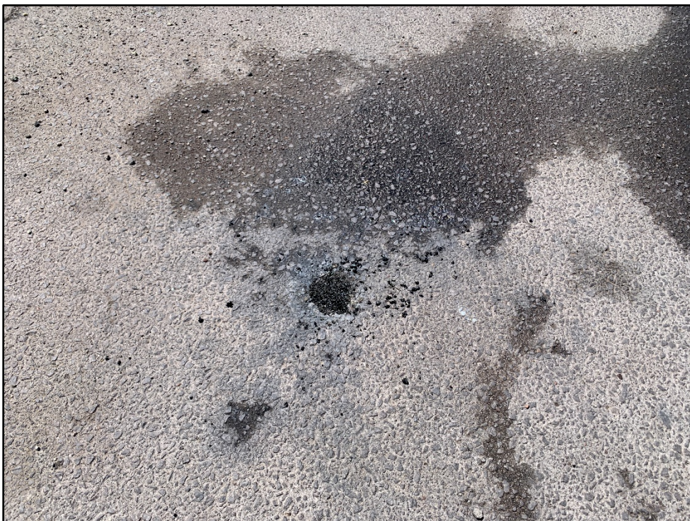
Photo 8. Plugged injection borehole.
