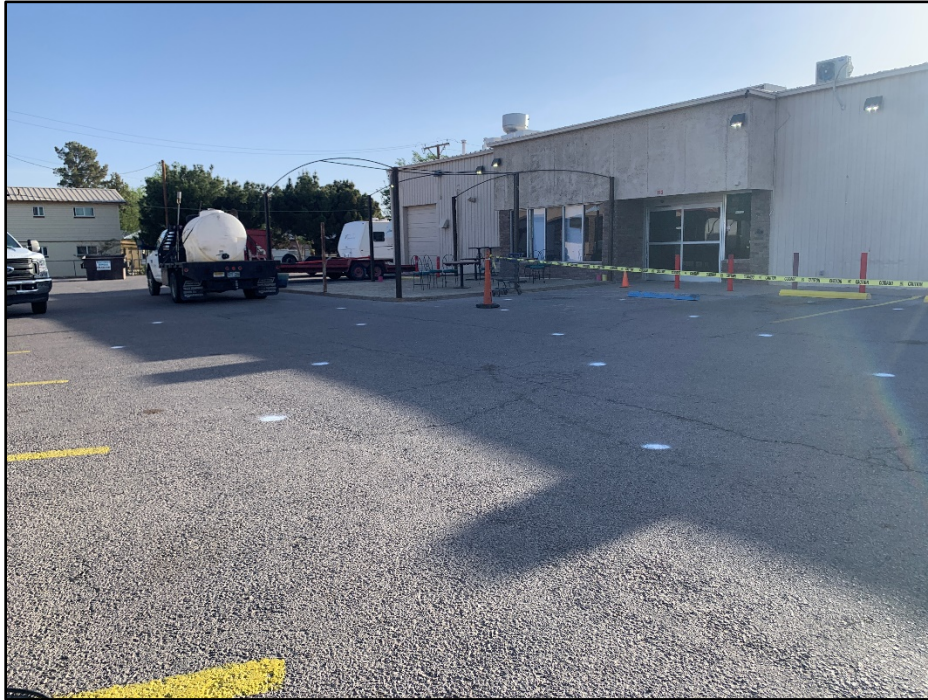
Photo 1. Pre-marked injection locations.
