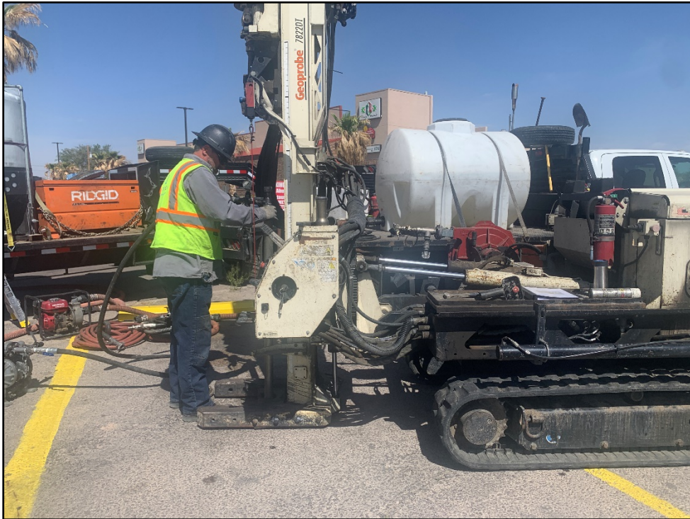
Photo 5. Drilling via direct push with Geoprobe.
