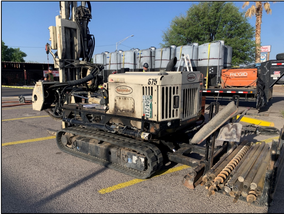
Photo 3. Geoprobe 7822DT and containers of 12% COGAC™ solution.
