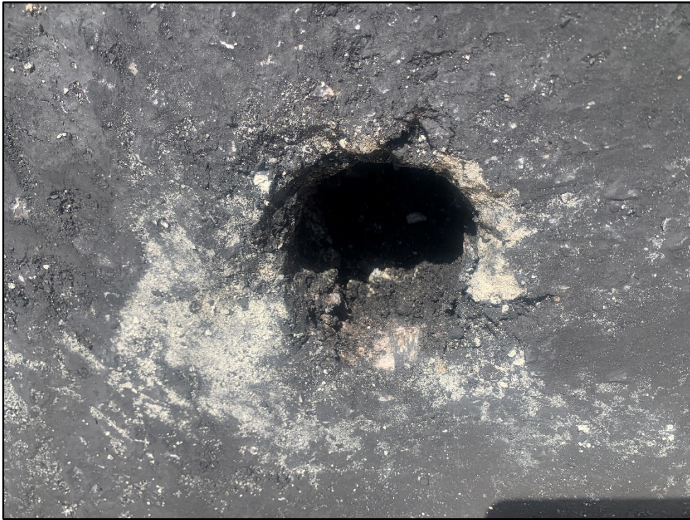
Photo 7. Injection borehole prior to plugging.
