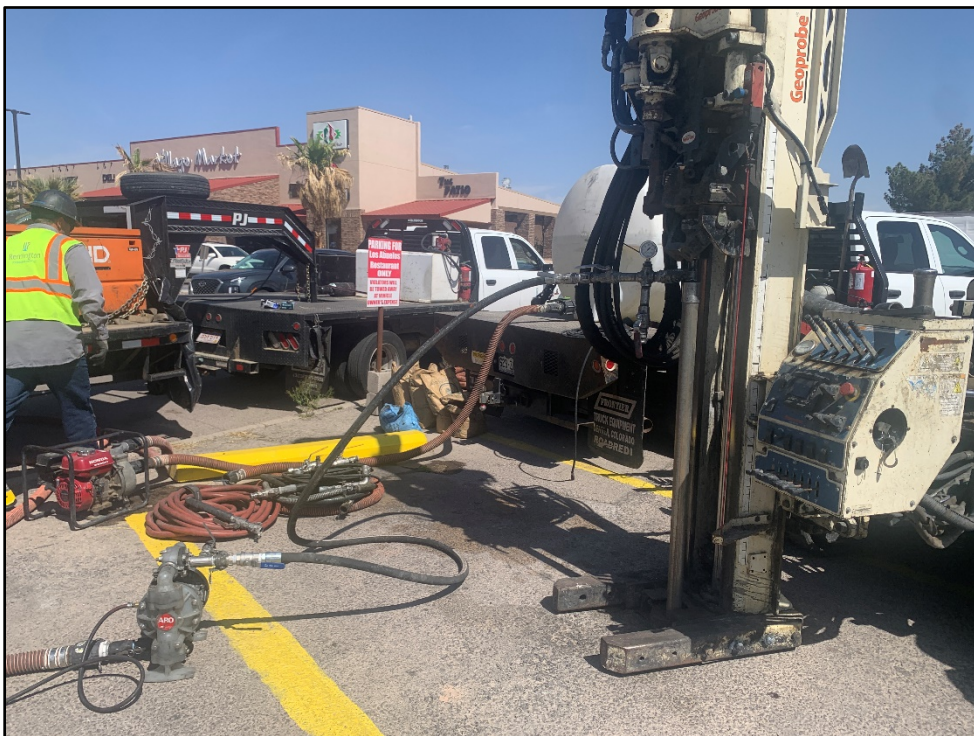
Photo 6. Injection of COGAC™ solution.
