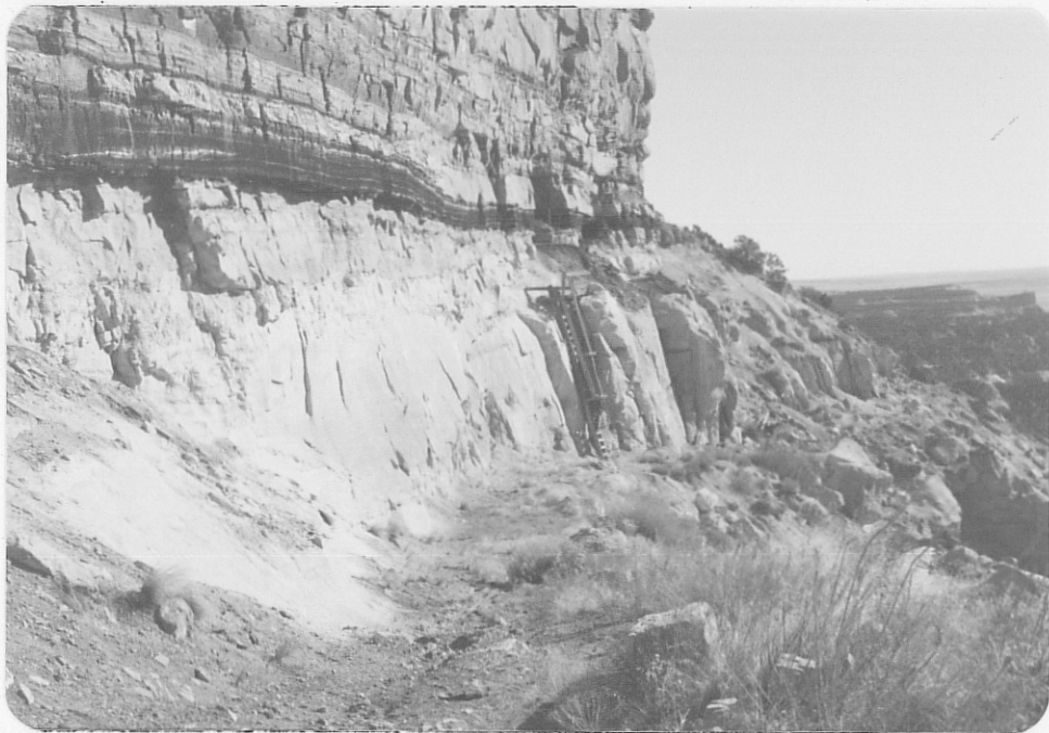
Photo (b) Looking east at ladder leading to Santa Fe Christensen adits (circled). The ore chute (lower circle) is just to the right of the ladder.
