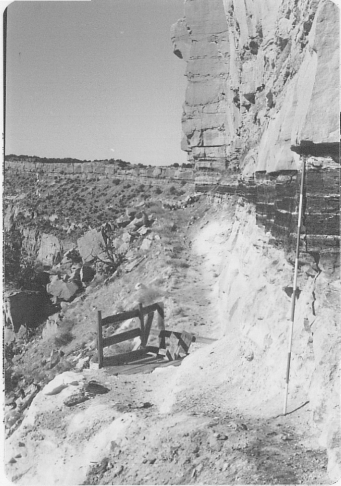
Photo (a) Looking west at access to the Santa Fe Christensen. Note wooden platform in foreground, and Christensen adit circled in background.
