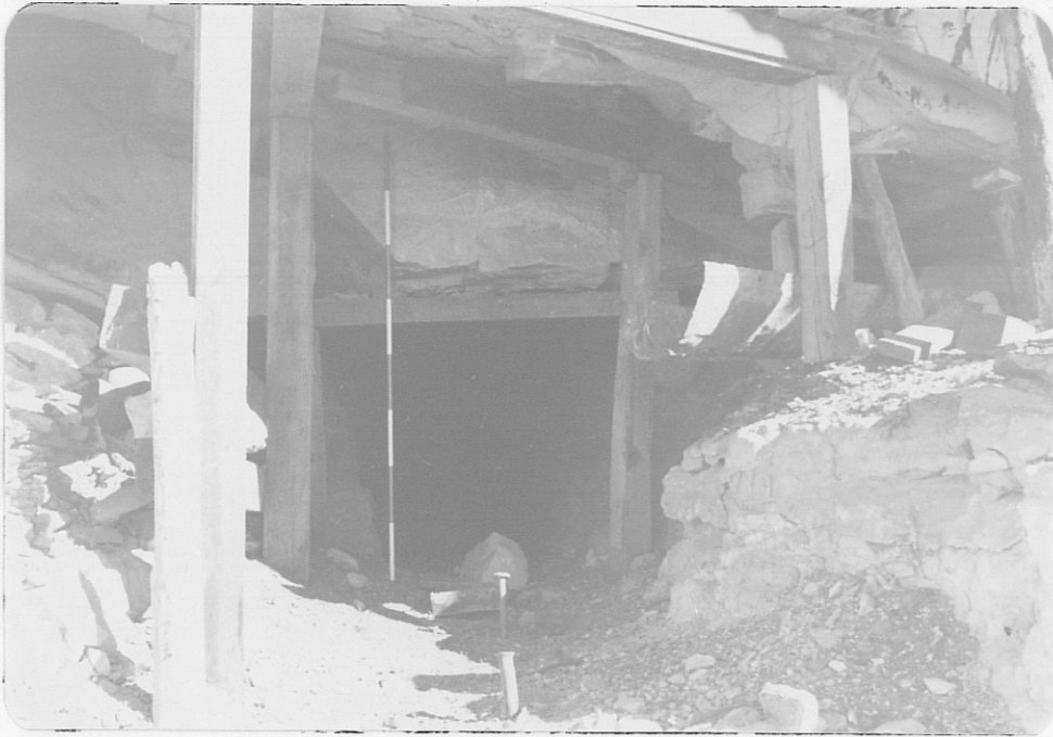
Photo (c) Looking NE at westernmost adit of the Santa Fe Christensen workings.
