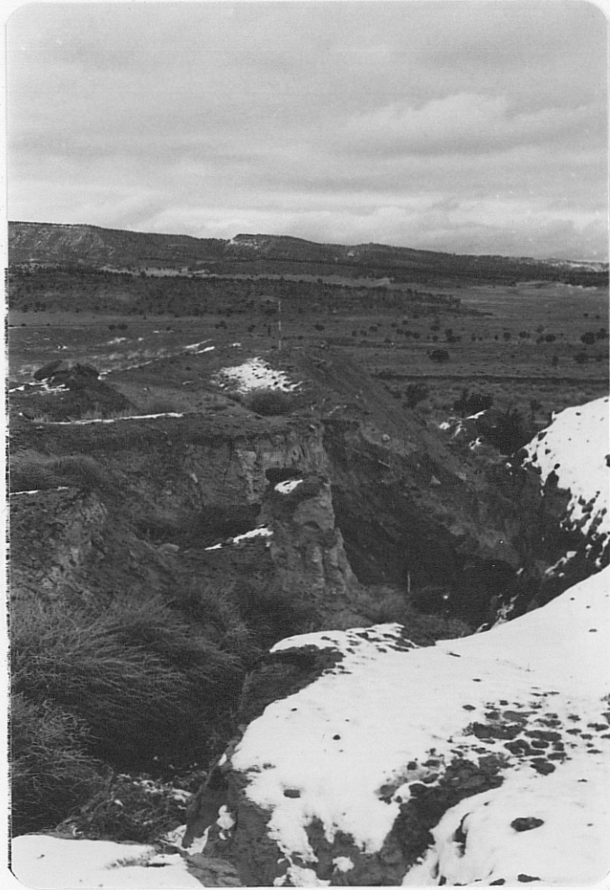
Photo (i) View northward at east edge of dump showing gullying; note range pole for scale and tributary in background visible through the gully notch.
