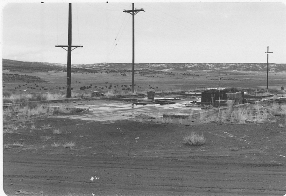
Photo (f) Looking northeastward at concrete slab and hoist and drum foundation. Slab measures 38' x 115'; note range pole for scale.
