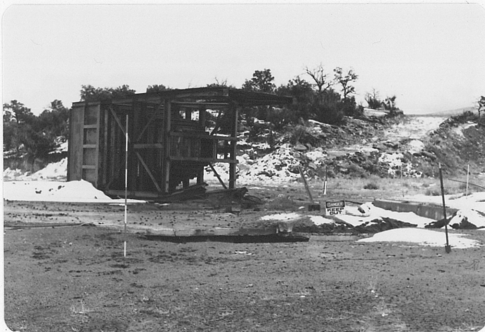
Photo (b) Looking northeast at shaft site showing caving which has begun around perimeter of concrete slab, and toppled ore bin; note range pole for scale.
