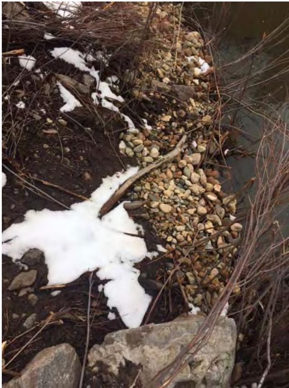
Photo 12 Backfill of Area #5 with river rock.
