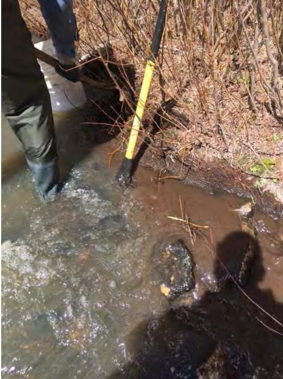
Photo 2 Removal of soil at Area #2 using hand tools.
