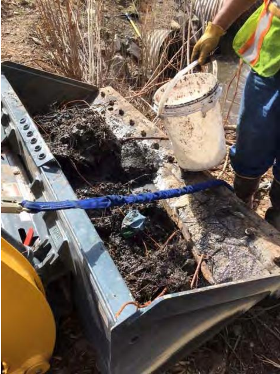
Photo 5 Use of bobcat to transfer soils to rolloff boxes.
