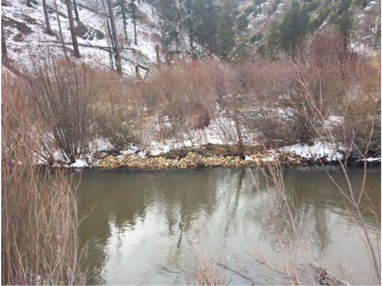
Photo 11 Backfill of Area #4 with river rock.
