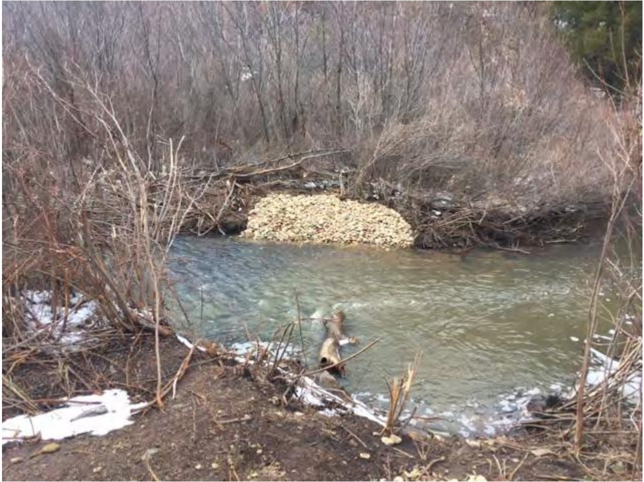
Photo 8 Backfill of Area #1 with river rock.
