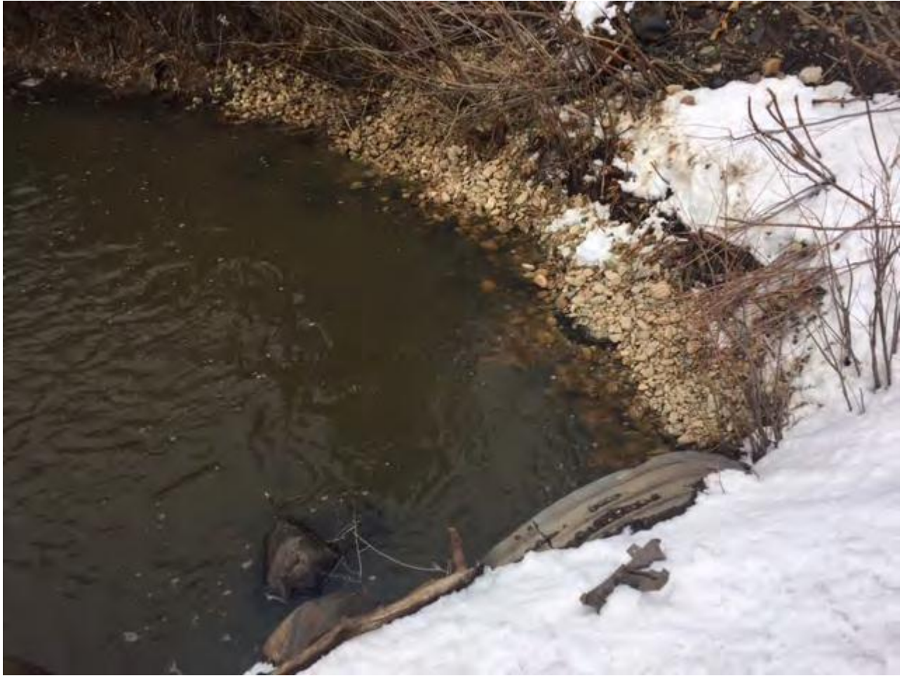
Photo 10 Backfill of Area #3 with river rock.
