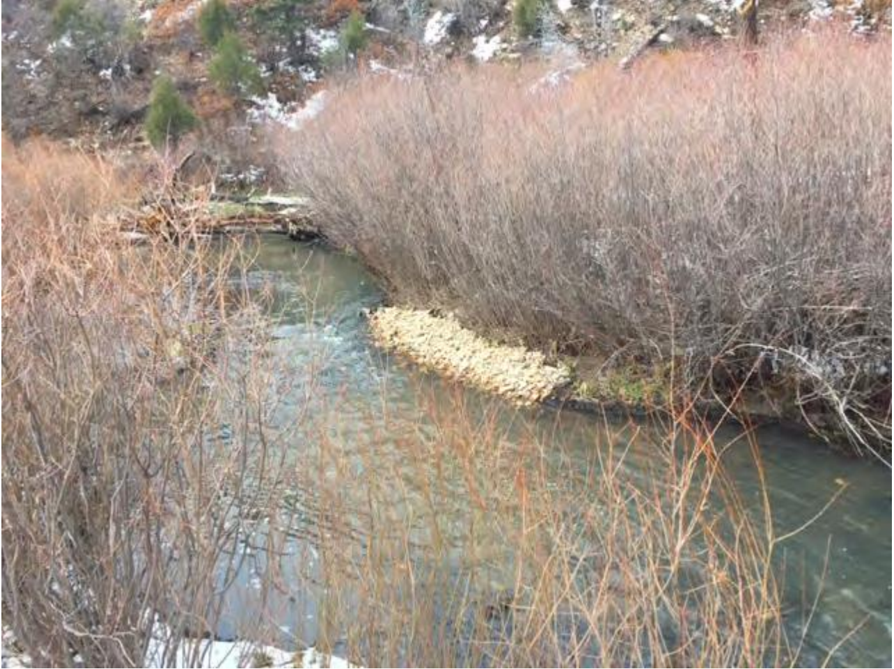
Photo 9 Backfill of Area #2 with river rock.
