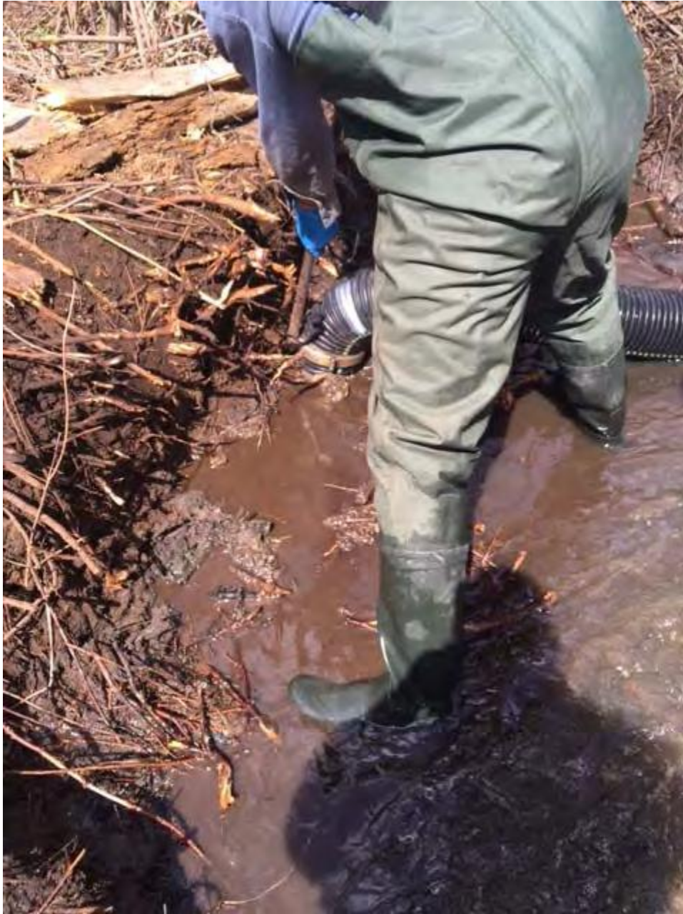
Photo 1 Removal of soil by Dry Vac truck at Area #1.
