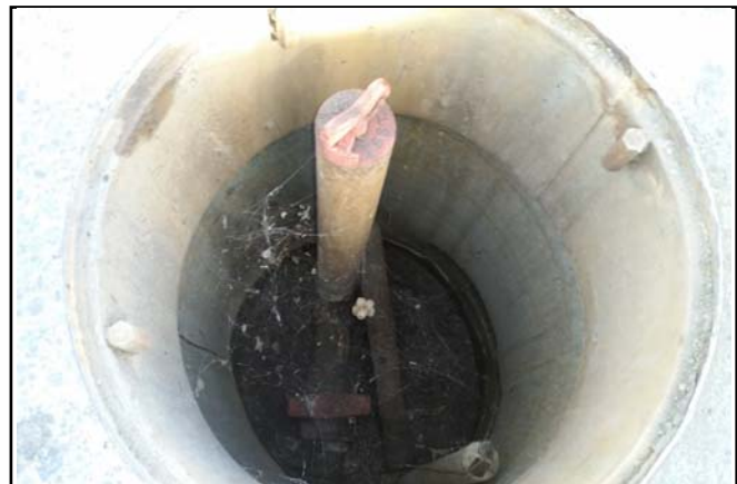
Picture 12 - Looking down into VP-2 well vault.
