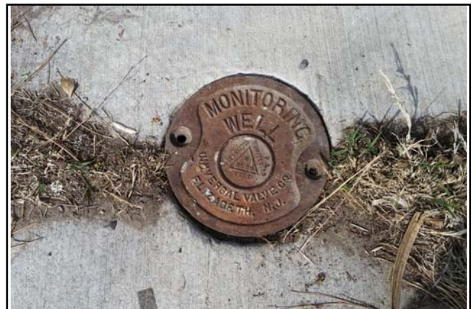
Picture 6 - Looking down at MW-7 well vault. Well vault cap is loose on concrete.
