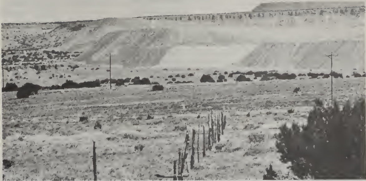
FIGURE 2-4 WASTE DUMPS ON NORTH SIDE OF MINE
