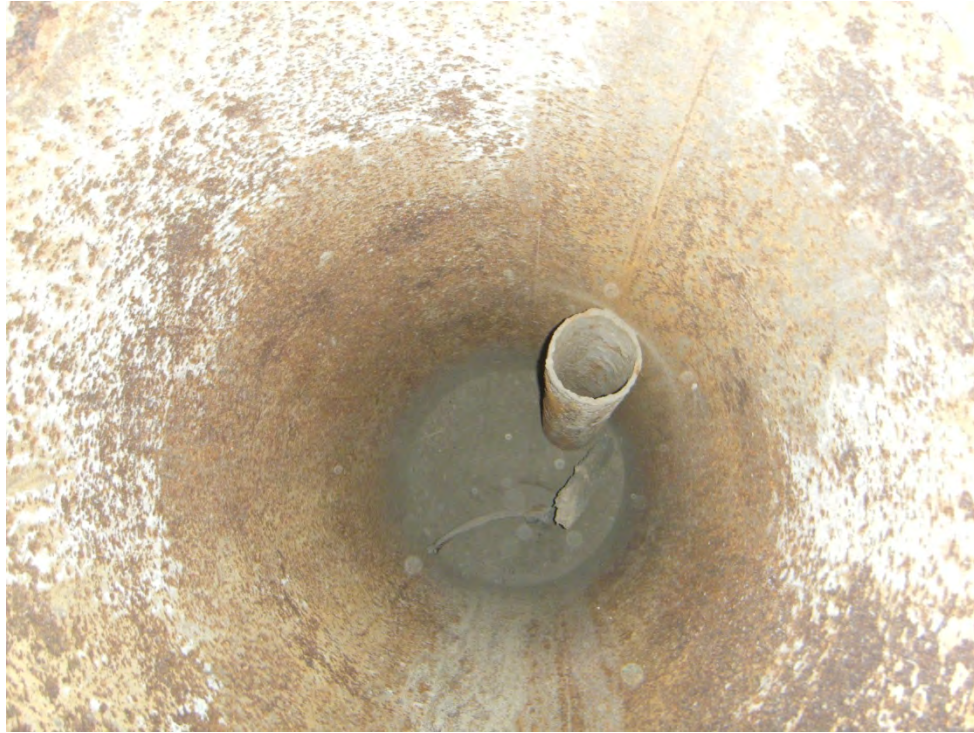
Photo 5-View down vent shaft (MiscPt-1).
