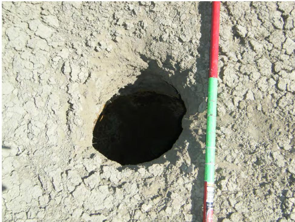
Photo 4-A vent shaft (MiscPt-1) in DistPly-1.
