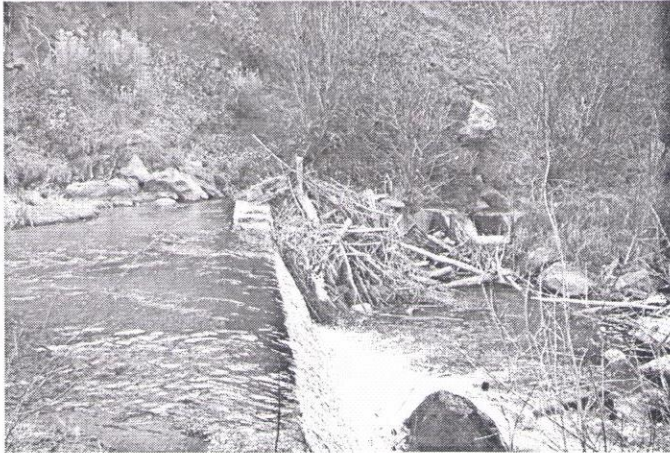
Diversion structure obstructing fish passage
