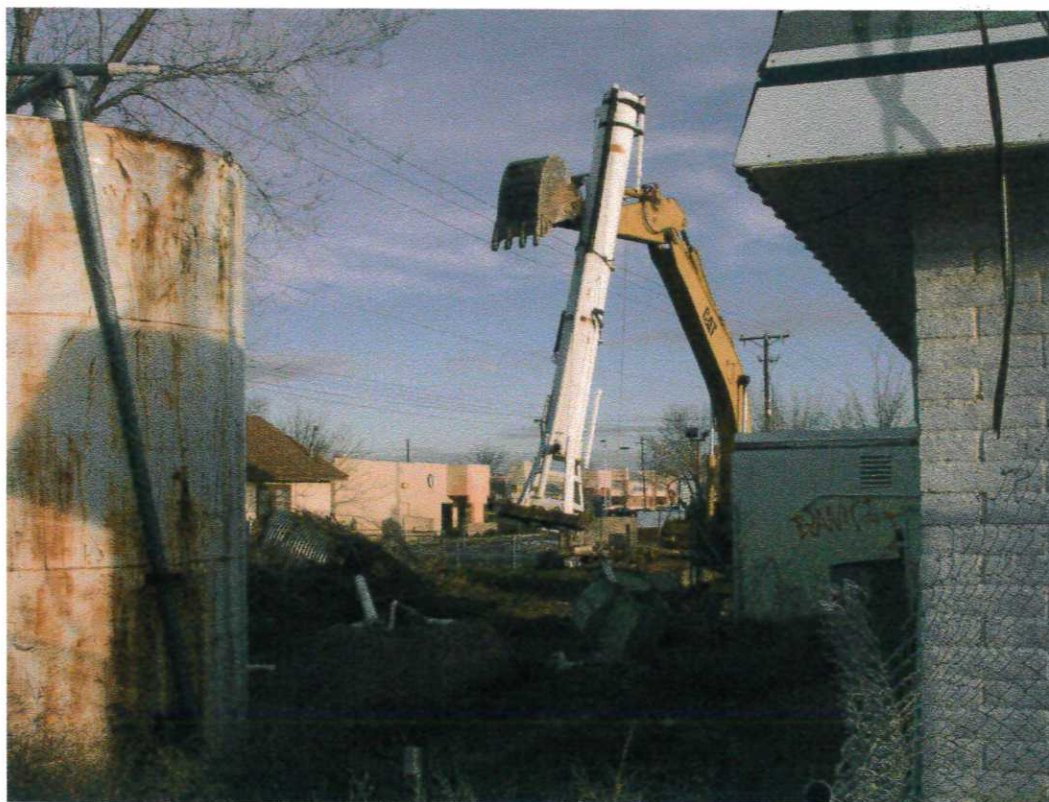
Photo 4. Removal of air stripper tower.
