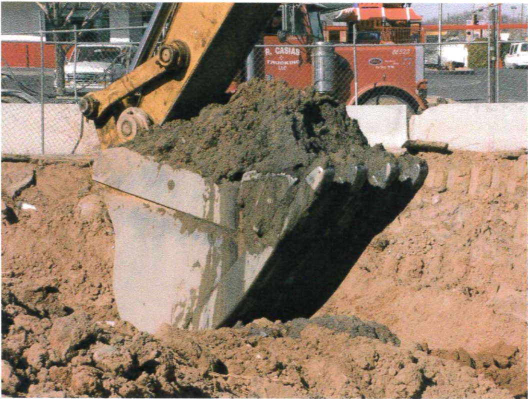
Photo 7. Removal of contaminated soil
