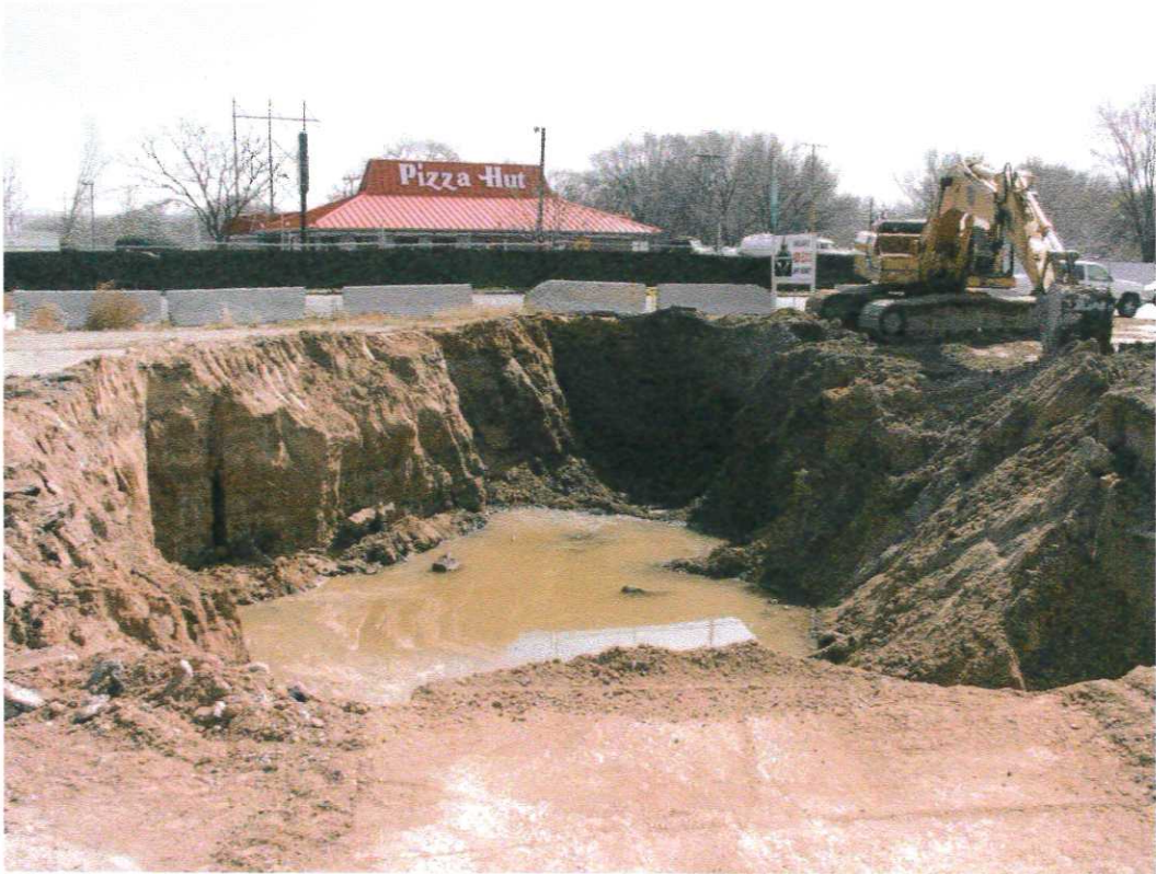
Photo 10. Continued removal of contaminated soil at north end of excavation area.
