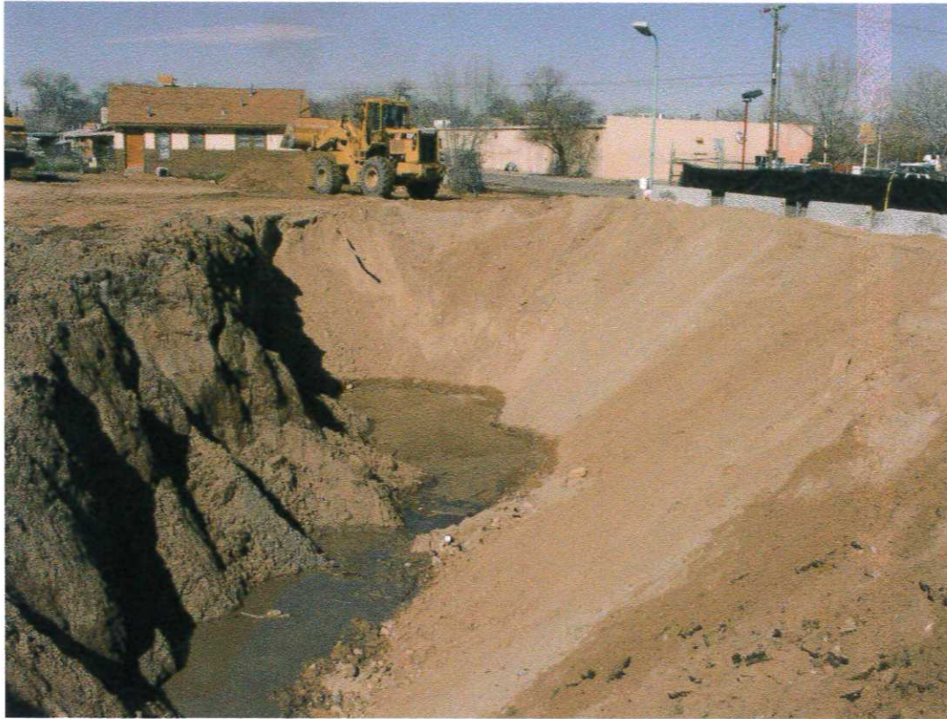
Photo 13. Backfilling with clean gravel and sand as the excavation moves southward.
