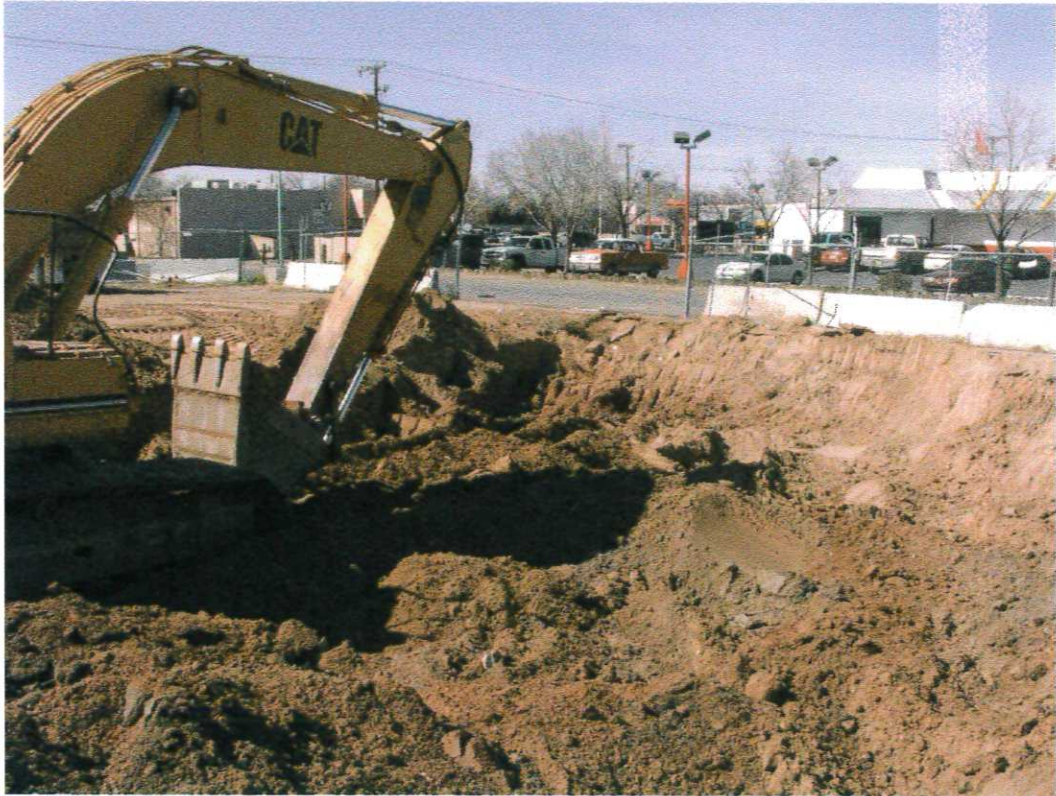
Photo 6. Continued removal of clean overburden.
