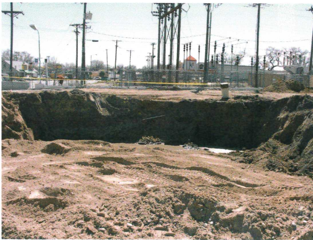
Photo 16. Excavation area looking south with clean backfill in the foreground.
