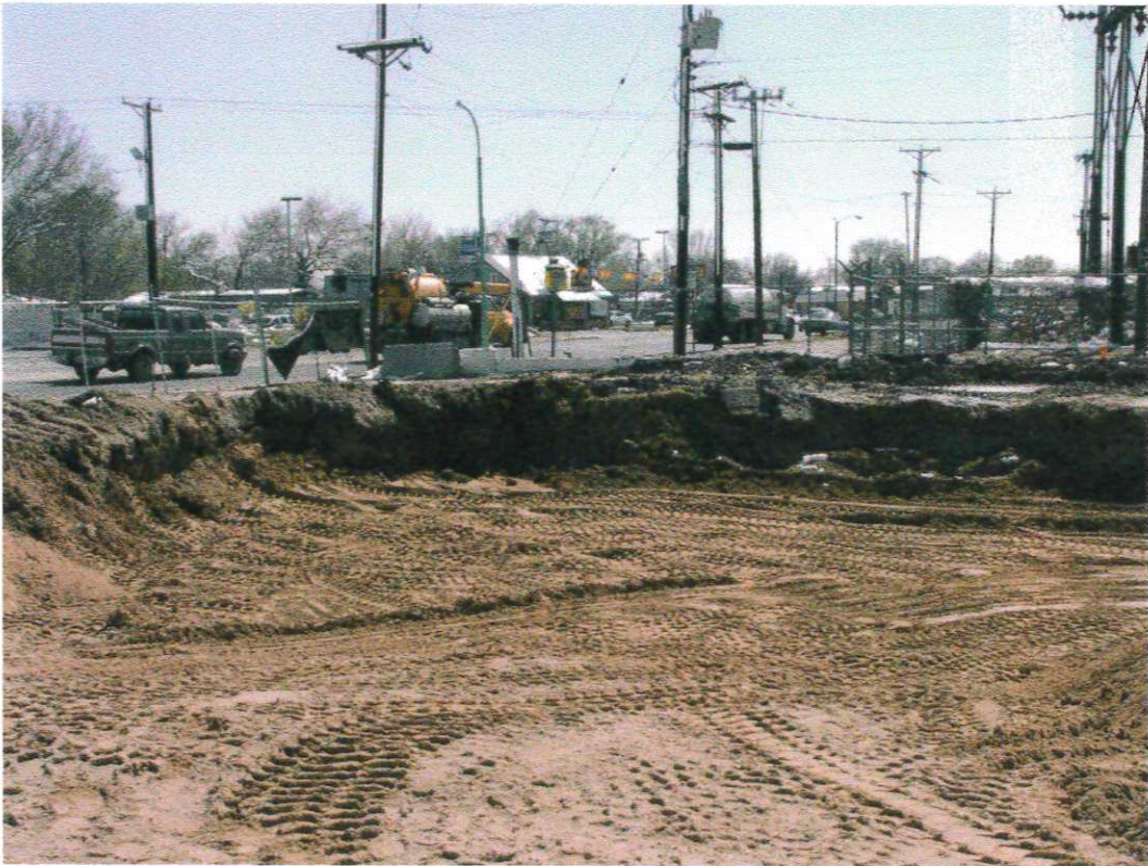
Photo 19. Backfilling and compaction of the excavated area.
