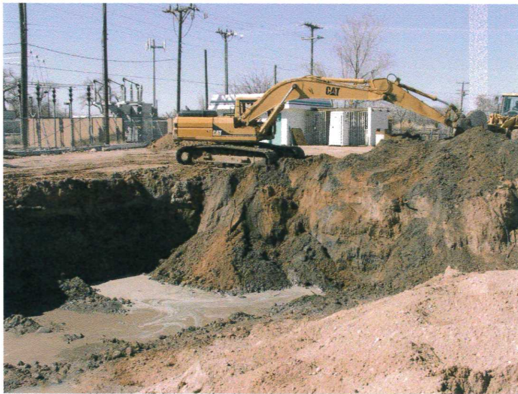
Photo 14. Removal of contaminated soil at southwest corner of excavation area.
