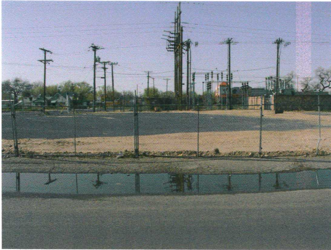
Photo 21. Restored site with crusher gravel over excavated area.
