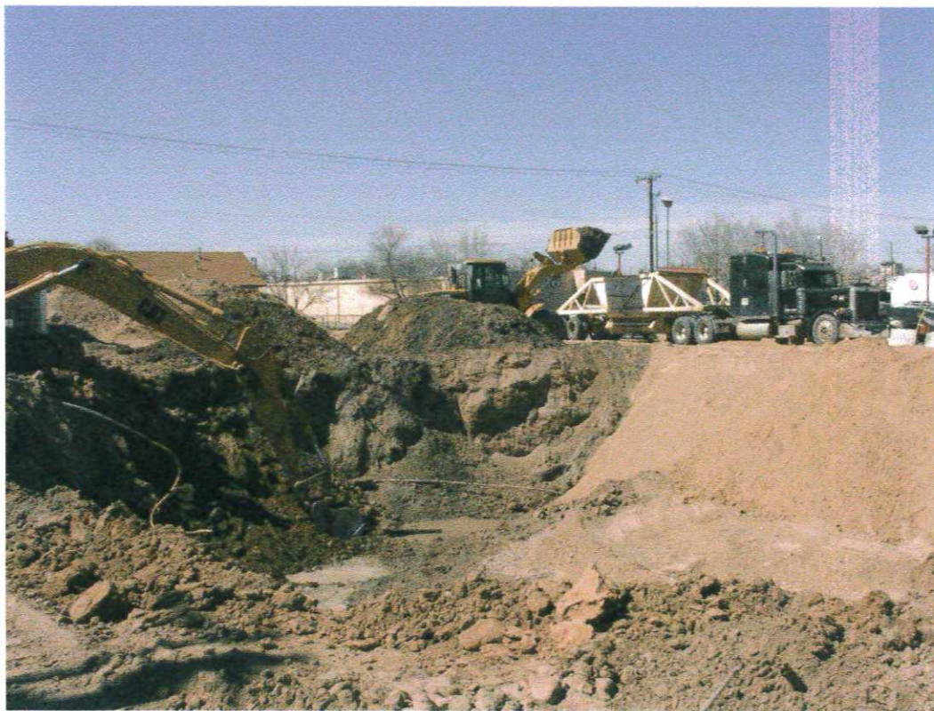
Photo 12. Loading contaminated soil into belly dumps
