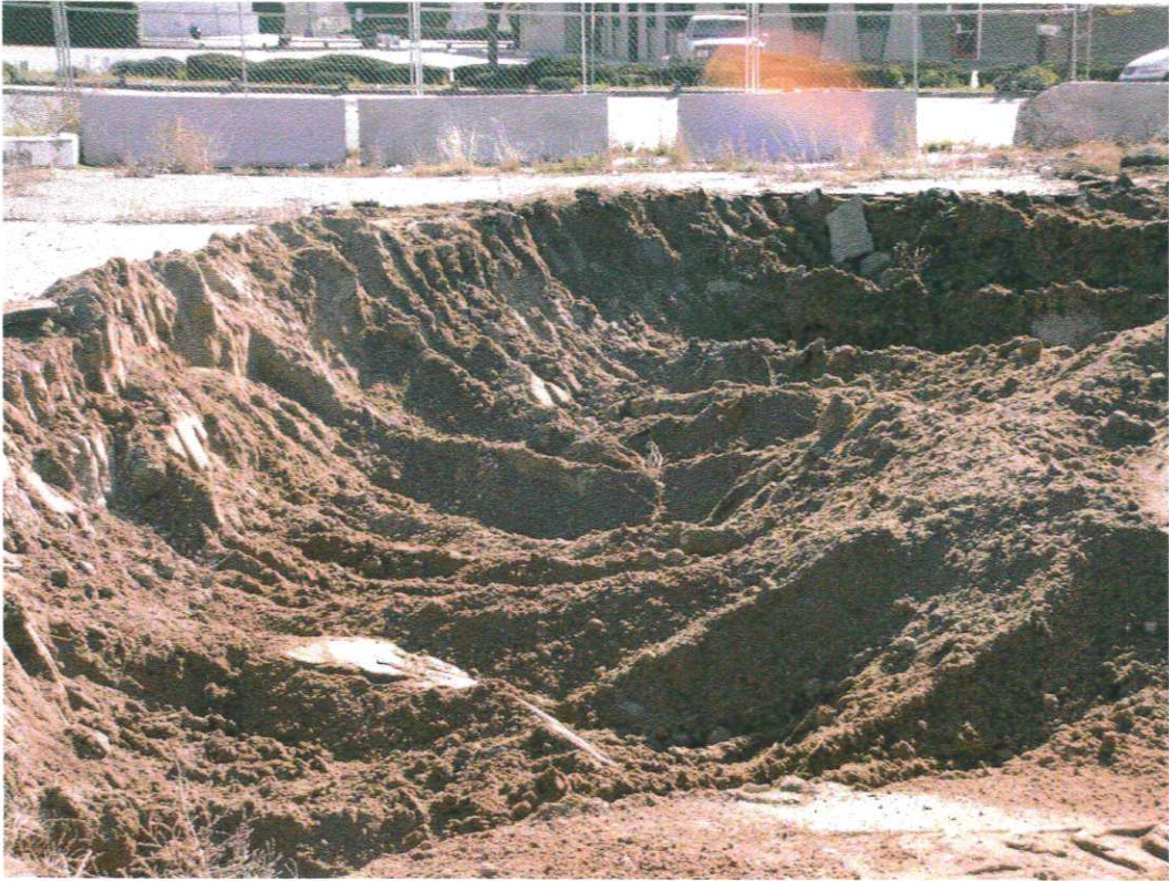
Photo 5. Removal of clean overburden on north end of excavation.
