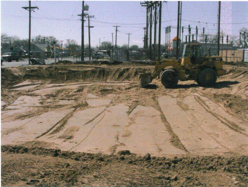
Photo 20. Continued backfilling and compaction of the excavated area.
