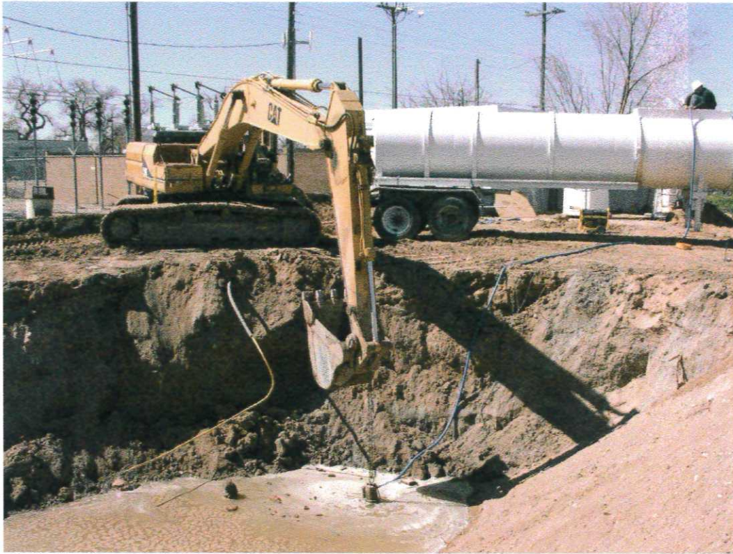
Photo 17. Removal of contaminated groundwater and a small amount of NAPL.
