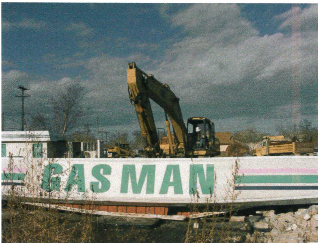
Photo 1. Demolition of canopy and pay booth.
