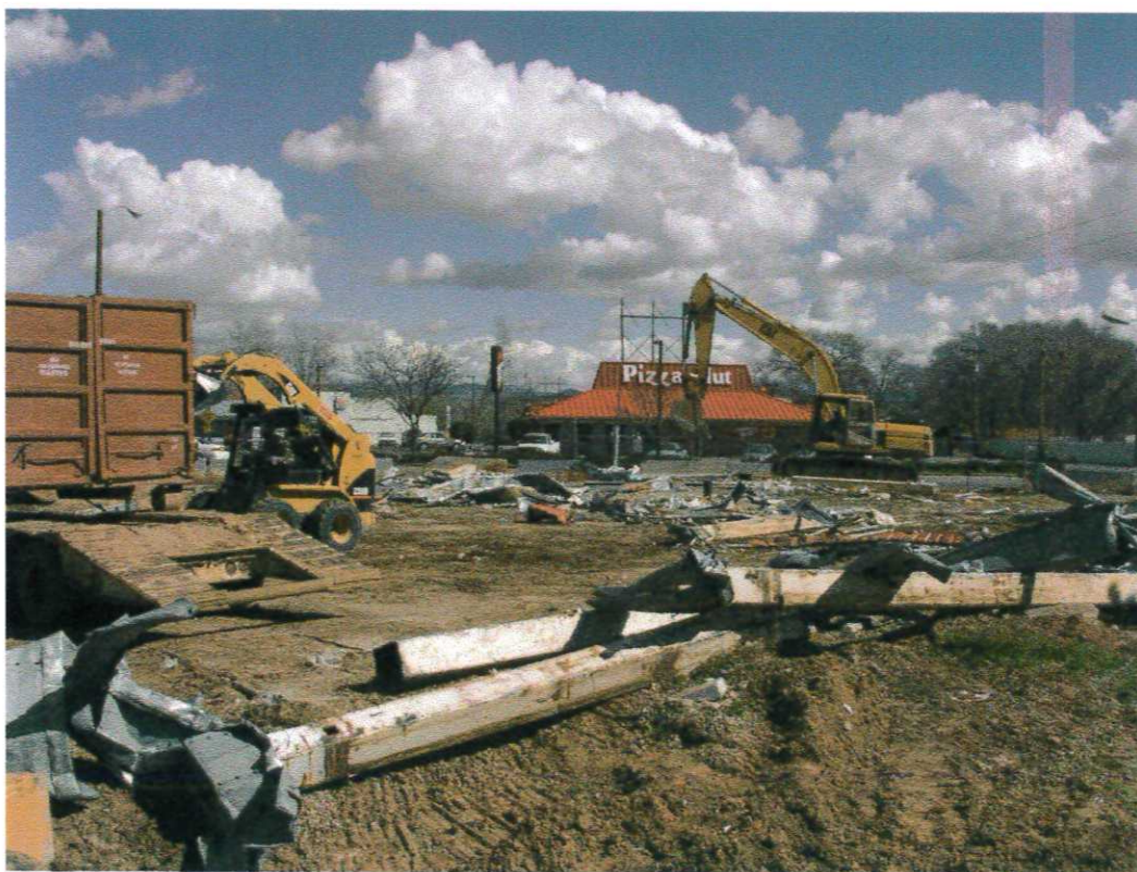
Photo 2. Demolition of canopy and pay booth.
