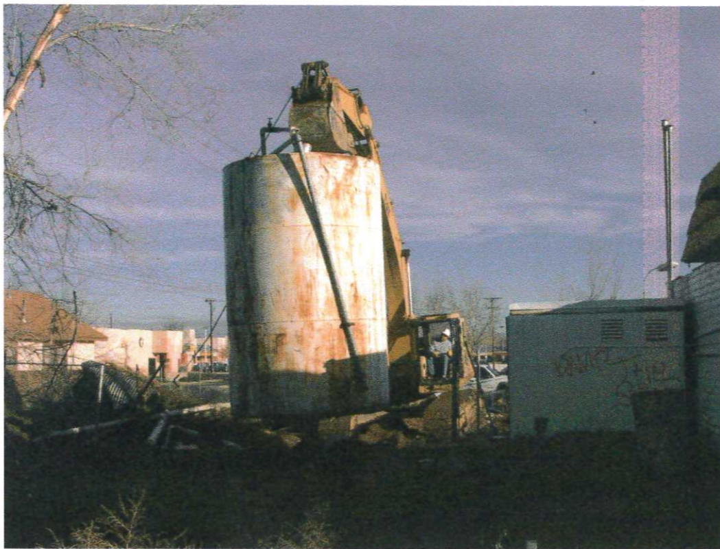
Photo 3. Removal of steel above ground influent settling tank.
