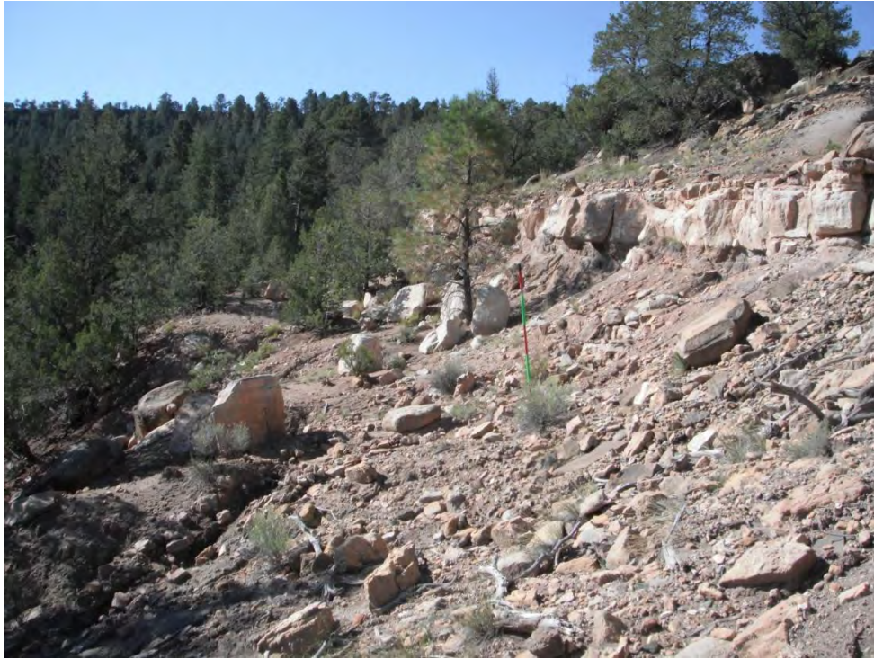
Photo 3-Looking southwest at CutLn-1, replicating Anderson photo C.
