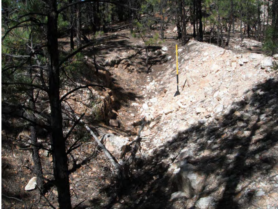
Photo 5-Looking west at Trench-1.
