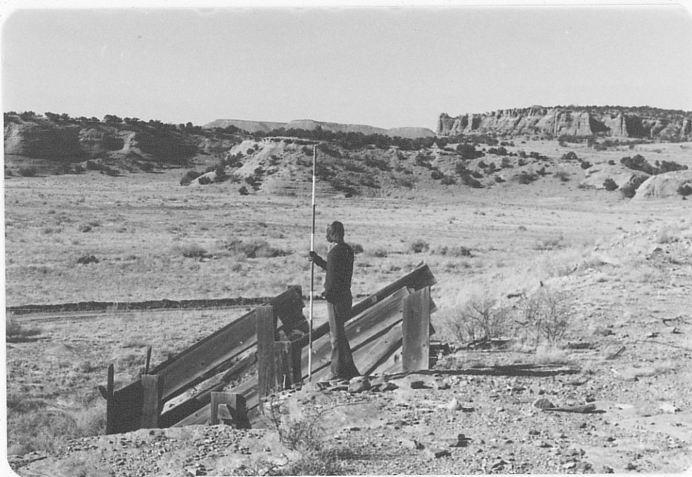
Photo (b) Looking NW at ore chute from access road level.
