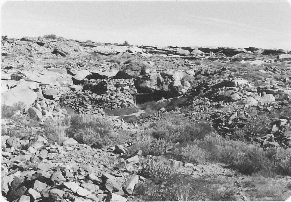
Photo E - King Tutt Point, looking NE toward eastside adit; portal about 5' high, 8' wide.
