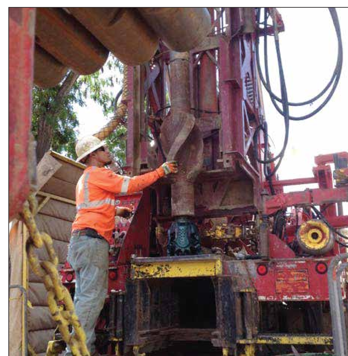
Well 234 Driller inserting bit into well
