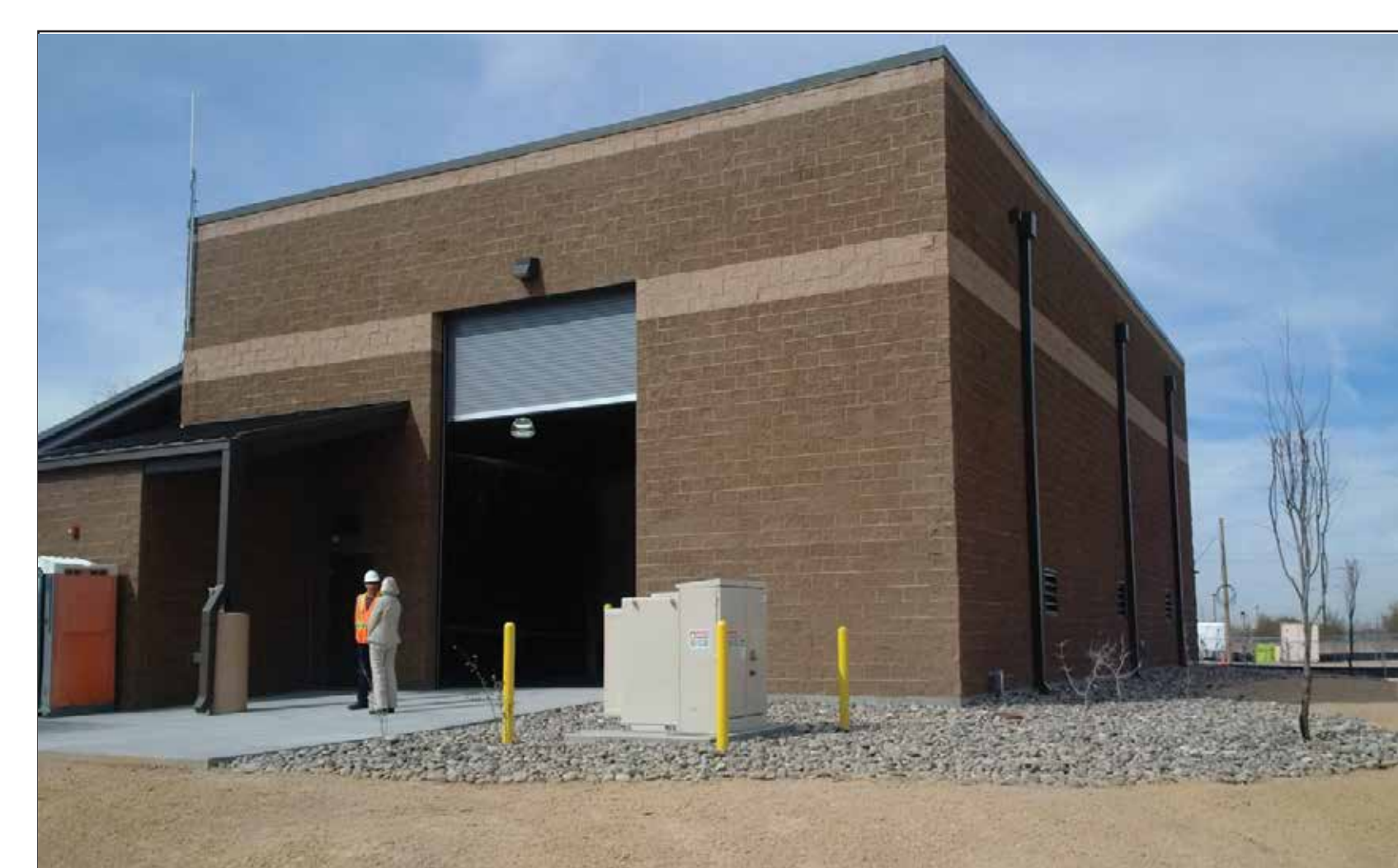
The GWTS began operation on December 31, 2015 with all three extraction wells. The full-scale GWTS consists of an influent holding tank, bag filters, two-20,000 pound vessels containing granular activated carbon, and a treated water storage tank.
