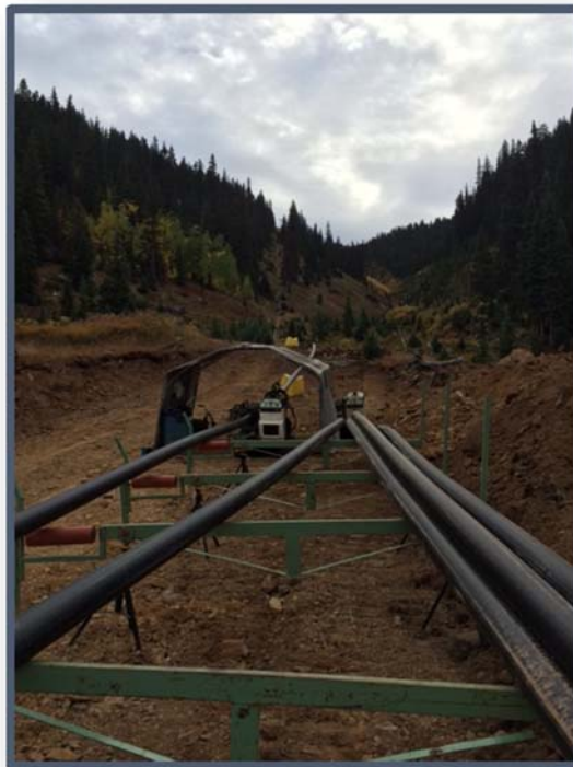
Installation of discharge piping downgradient of Gold King Mine
