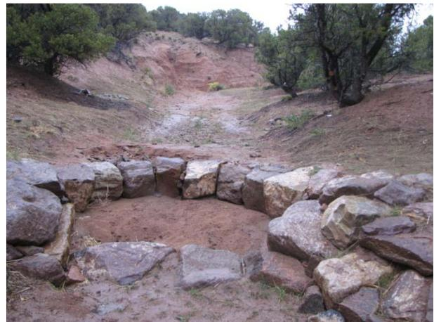
**Figure 4.7.** (Left): One-Rock-Dam and rock rundown in Arroyo Saiz in Santa Fe (looking upstream). Photo by Earth Works Institute 2010.
