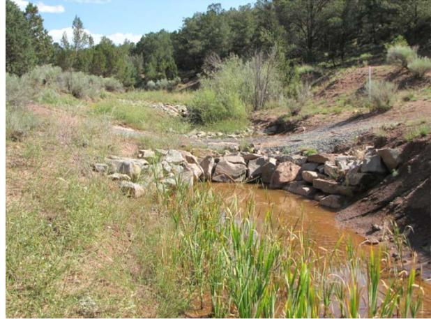
**Figure 4.5.** (Left): A series of rock cross vanes in Cañoncito Arroyo (Eldorado Community Preserve) wetlands raised the grade of the stream and made point bars, the flood plain and adjacent riverine wetlands accessible to lower level (more frequent) floods.
