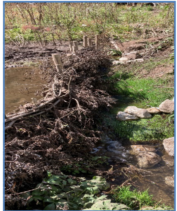
Above; Beaver Dam Analogues on Big Bear Creek show a lot of buildup of sediment upstream of the structures only six weeks after installation.
