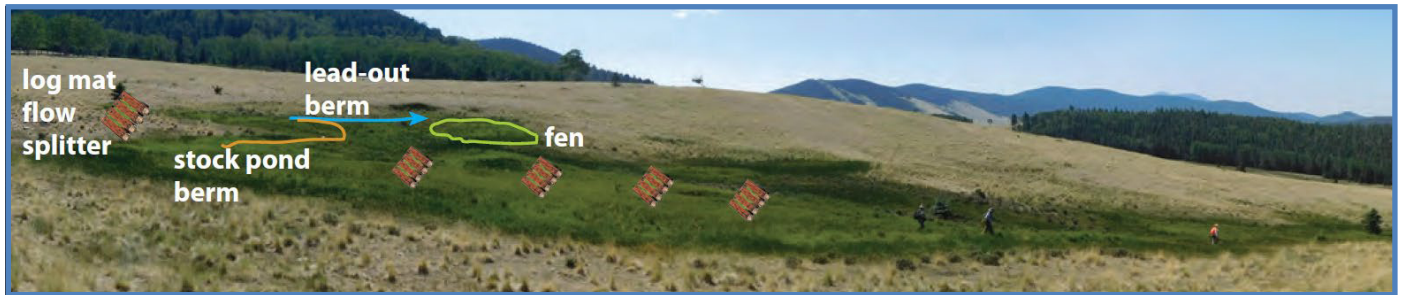
Figure 18. A schematic overlay from the Technical Guide shows on a treatment train in Middle Holman Creek. Water is continually spread from the main channel to wetland surfaces to enhance infiltration and storage. Blue arrow indicates flow direction. Green polygon is a fen. Log icons indicate locations of restoration structures.
