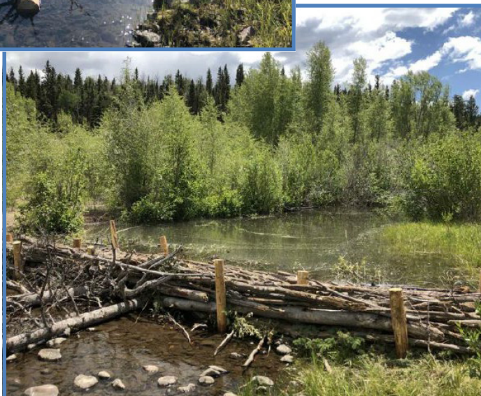
Photo above; Rio San Antonio post-assisted log structures from 2020.
