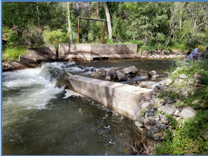
Photo above left; Old diversion dam structure.
