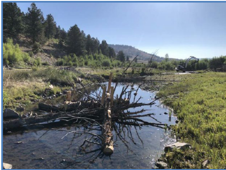
Photo above; Rio San Antonio post-assisted log structures from 2020.
