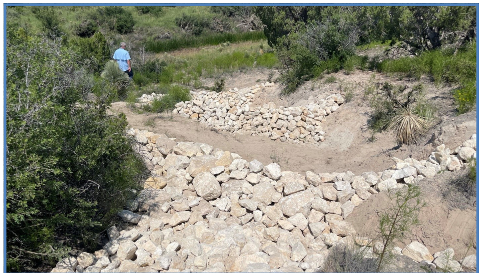
Completed check dams near the Black River.
