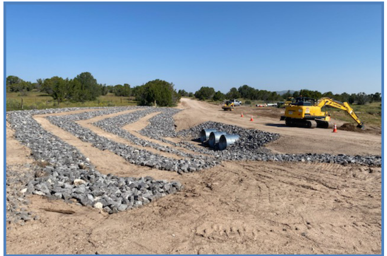
Reconstructed road crossing on unnamed tributary of Arroyo Montosa
