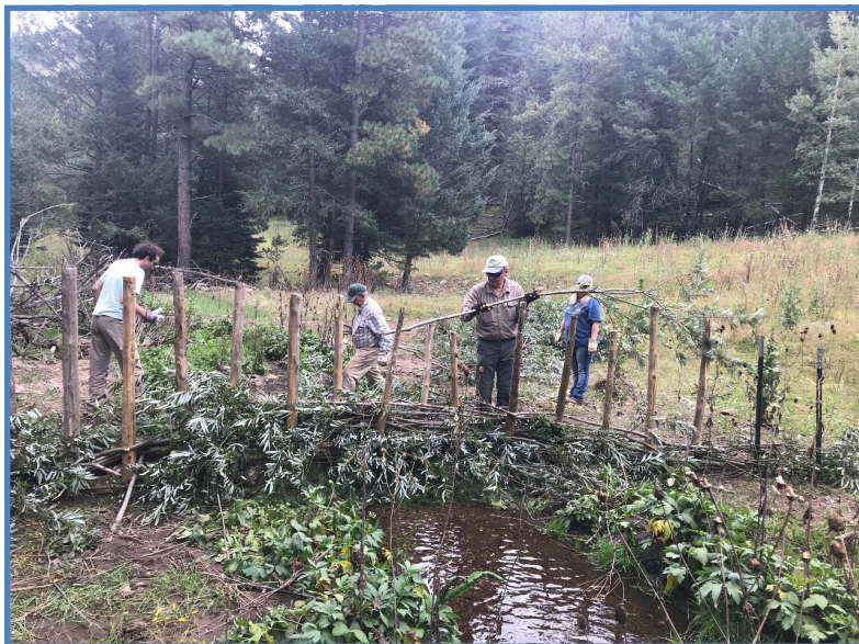
Above; Beaver Dam Analogues on Big Bear Creek show a lot of buildup of sediment upstream of the structures only six weeks after installation.
