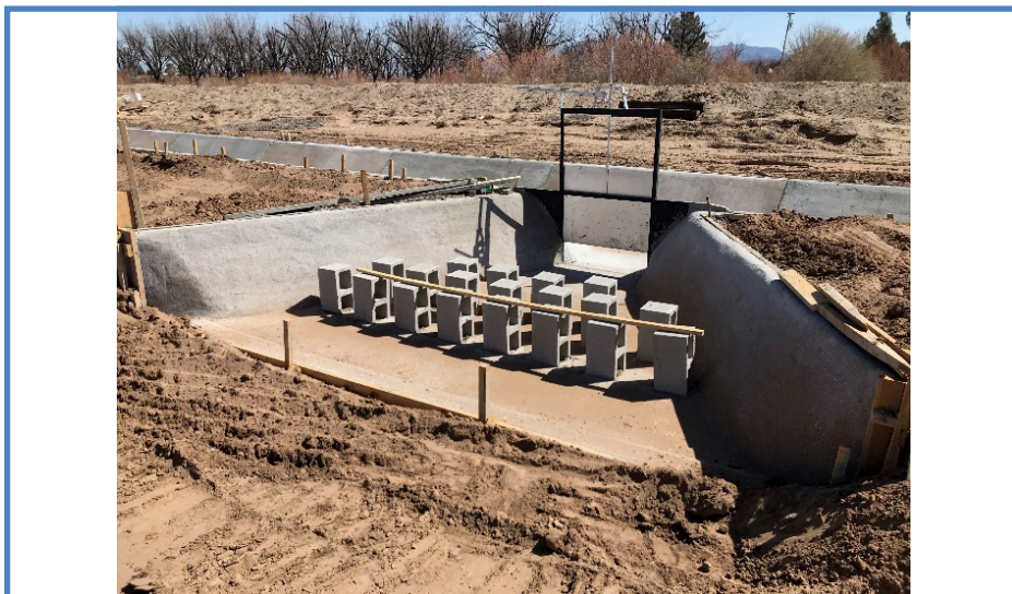
Lined Ditches and Structures for Water Control installed through the NWQI.
