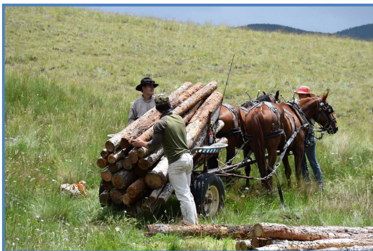
Figure 19. Logs were hauled via horse drawn trailer for log structures during the August 2019 volunteer workshop in the upper East drainage. One of the project challenges was getting the materials to the building sites. Horses could easily handle the terrain and the volunteers enjoyed watching them transport the logs.
