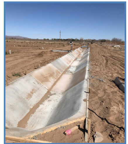
Lined Ditches and Structures for Water Control installed through the NWQI.
