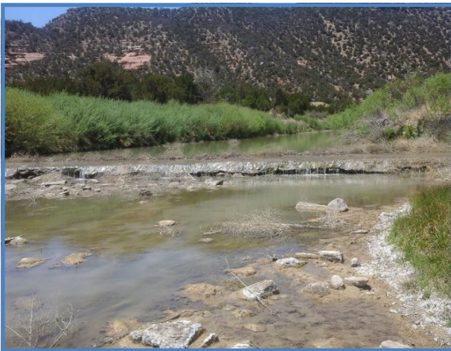
Low water crossing (looking upstream) in Mills Canyon, Canadian River before and after construction of the improved crossing completed in FY21 to provide passage for aquatic organisms.
