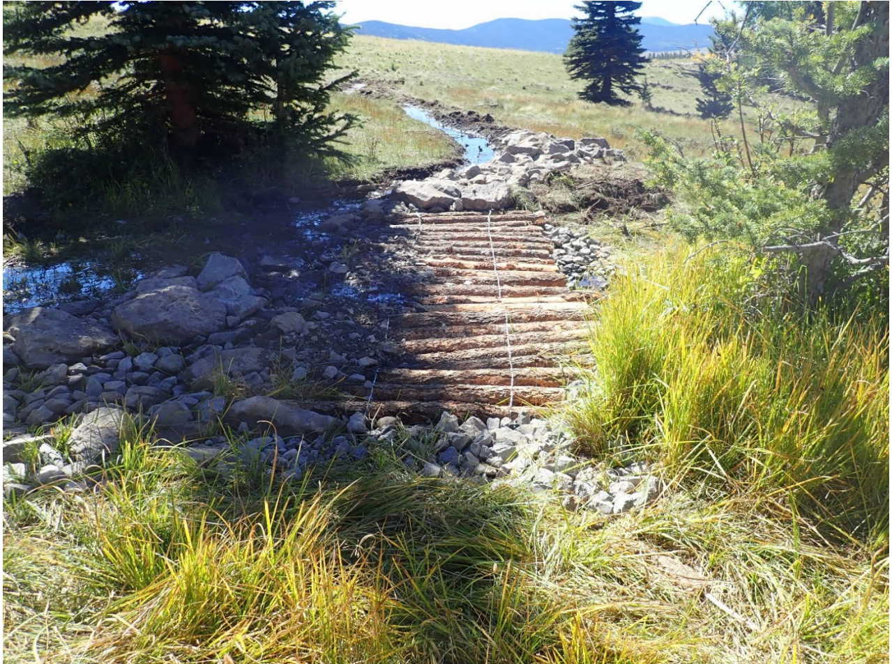
Log Split, Log Mat and Log Reinforced Contour Berm spreads water across a previous wetland surface, West Drainage, Holman Creek Watershed Complex. September 13, 2018. Photo by Emile Sawyer
