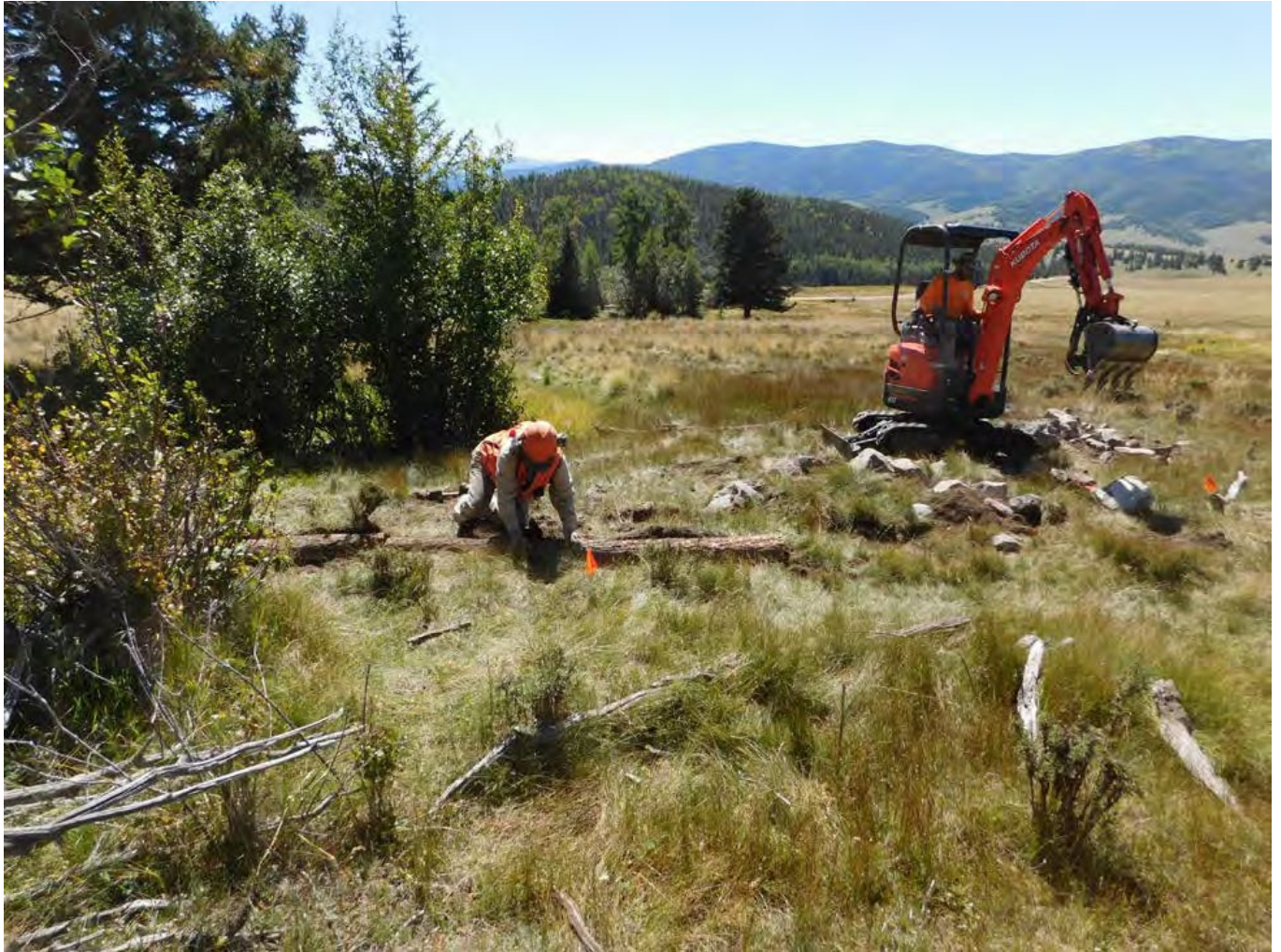
Figure 4. The mini-excavator is used to dig and place anchor rocks, while manual labor, shown here by Margie Tatro, is used to set and chink log berm structure. Photo by Mollie Walton.
