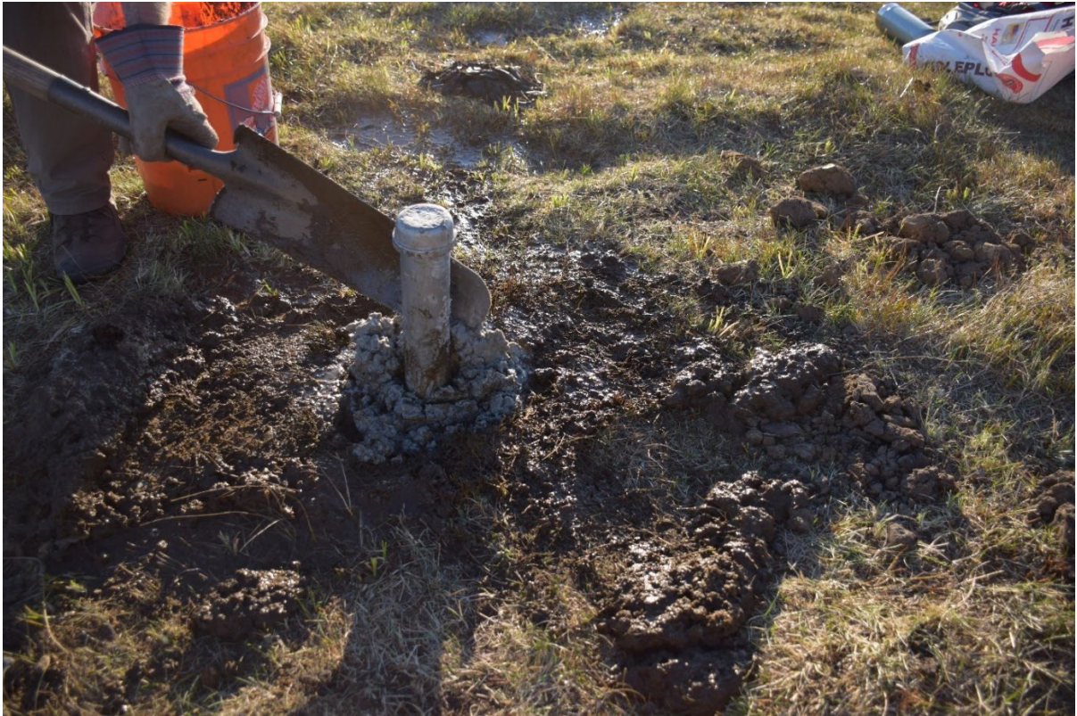
Figure 14. Gunner Johnson fills borehole with bentonite mixture to complete P6E2DS piezometer.
