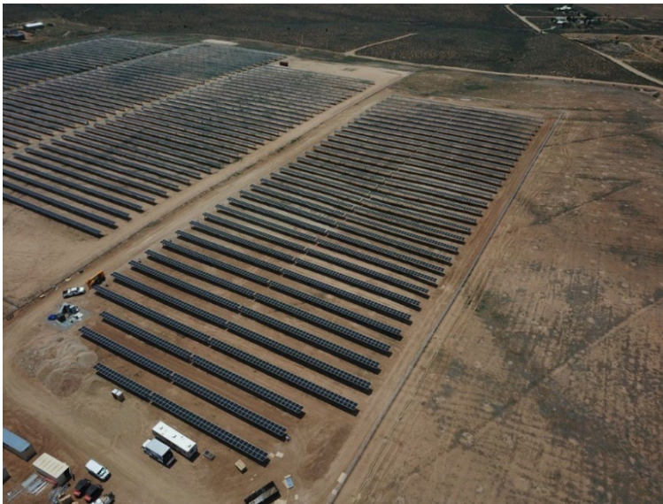
Solar Array for Taos Wastewater Treatment Plant CWSRF
