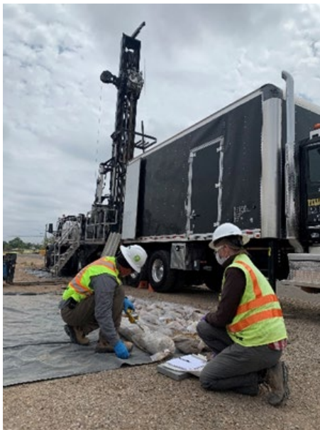
Observation of Groundwater Well Drilling
