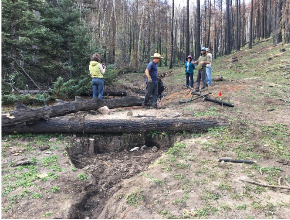
a) Post Fire Rehabilitation of the Rio en Medio: Volunteers stabilizing a gully to promote deposition of sediment onto an alluvial fan above the Rio en Medio.
