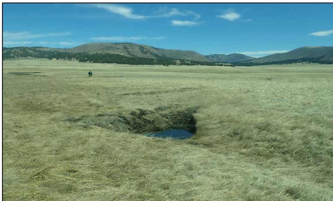
[Above] Excavator Plug structure in early spring after snowmelt. The water is flowing toward the person downslope.
