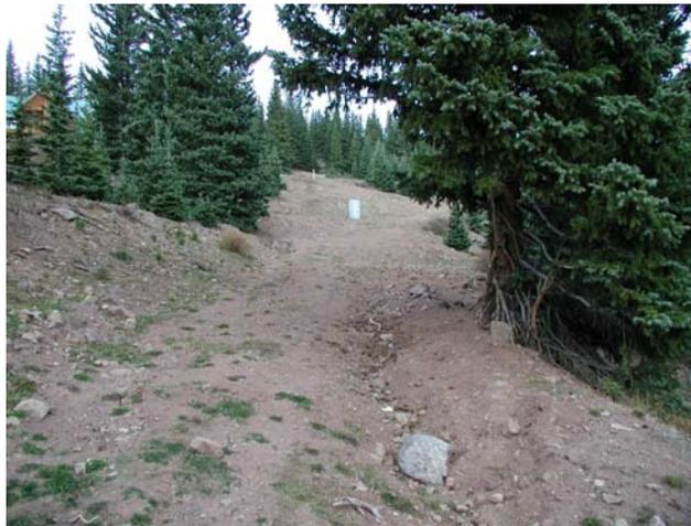
*Figure 13 Roads and Ski Runs Have Altered Drainage*
