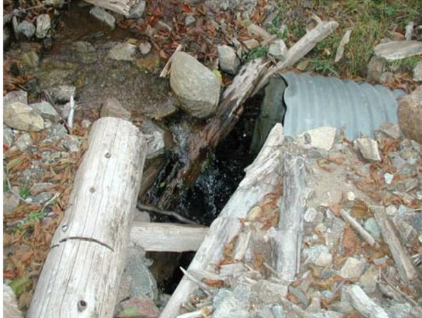
*Figure 12 Culvert Opening Almost Plugged*
