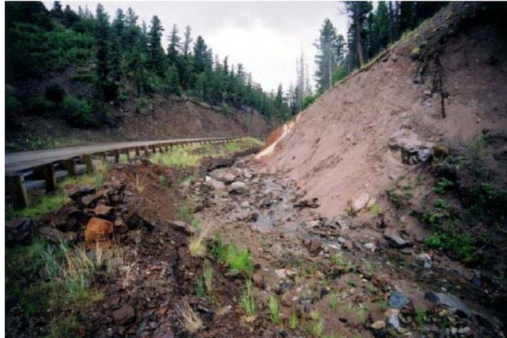
*Figure 14 Bank Erosion Along NM 196*
