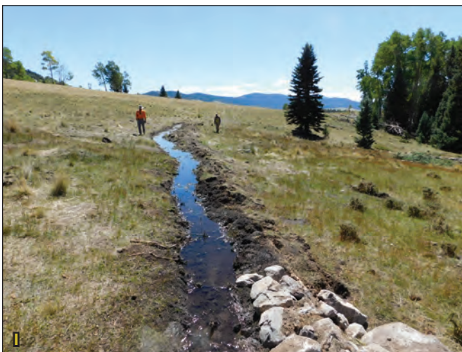
Figure 4.10I. One day after completion of the treatment train, water reaches the far end of the swale and berm structures. Figure 4.10J. After one year, the structures are saturating the former wetland downslope.
