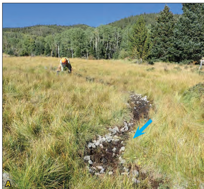
Figure 4.14A. This modified channel above was stabilized with rock armor. One rock dams were also installed as needed to further stabilize and aggrade the channel, while spreading sheet flows back onto the wetland surface. Figure 4.14B. This channel remained stable the following year. Sheetflow was re-established during snowmelt, restoring floodplain connectivity. Blue arrows indicate flow paths.
