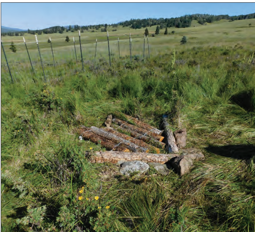
The above photo shows a log mat flow splitter (center) constructed to intercept channelized flow and convert it to sheetflow which will be intercepted by vegetation in the enclosure (fencing top left). Keyline Design principles lend themselves to linked treatment structures to maximize water spreading and harvesting benefits.
