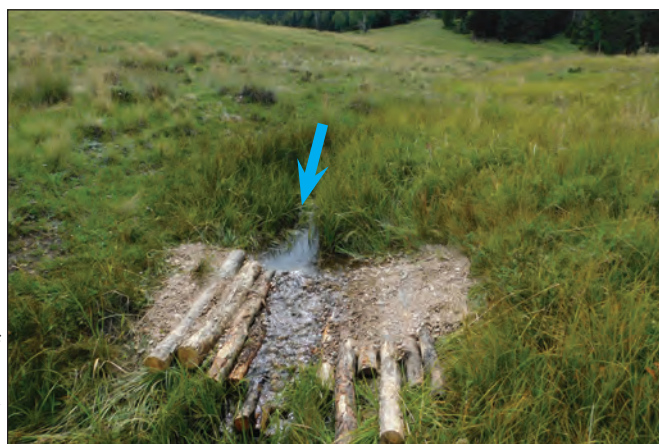
Figure 4.3. This log mat flow splitter was built upstream of a large headcut. It spreads the majority of flow to valley right through a rock and log reinforced lead-out berm. Existing vegetation was carefully incorporated into the flow splitting structure and new vegetation is colonizing the treatment area. The downstream area is kept saturated but the flow splitter prevents it from receiving erosive flows. Blue arrow indicates flow direction.
