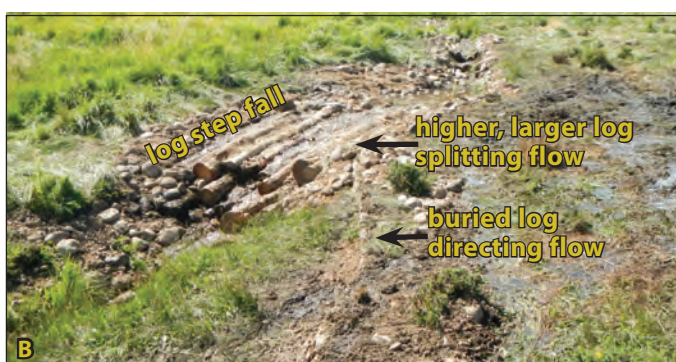
Figure 4.8A. A log step fall with flow splitter directs water from the channel to rehydrate a disconnected slope wetland area towards valley left. Blue arrows indicate flow paths. Figure 4.8B. This photo shows the same structure; built higher on valley left to direct flow downslope. Black arrows indicate flow direction across structure.
