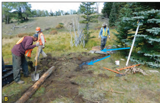
Figure 4.10A. The location for the log mat flow splitter was surveyed to ensure that water could be moved out of the channel at the proper elevation. Figure 4.10B. A swale was created to receive the water diverted from the channel by the log mat flow splitter. Figure 4.10C. The log structure diverts water to the swale. Figure 4.10D. A log mat is installed in the main channel below the flow splitter to raise the grade of the incised channel and further spread water over the wetland surface. Blue arrows indicate flow paths.
