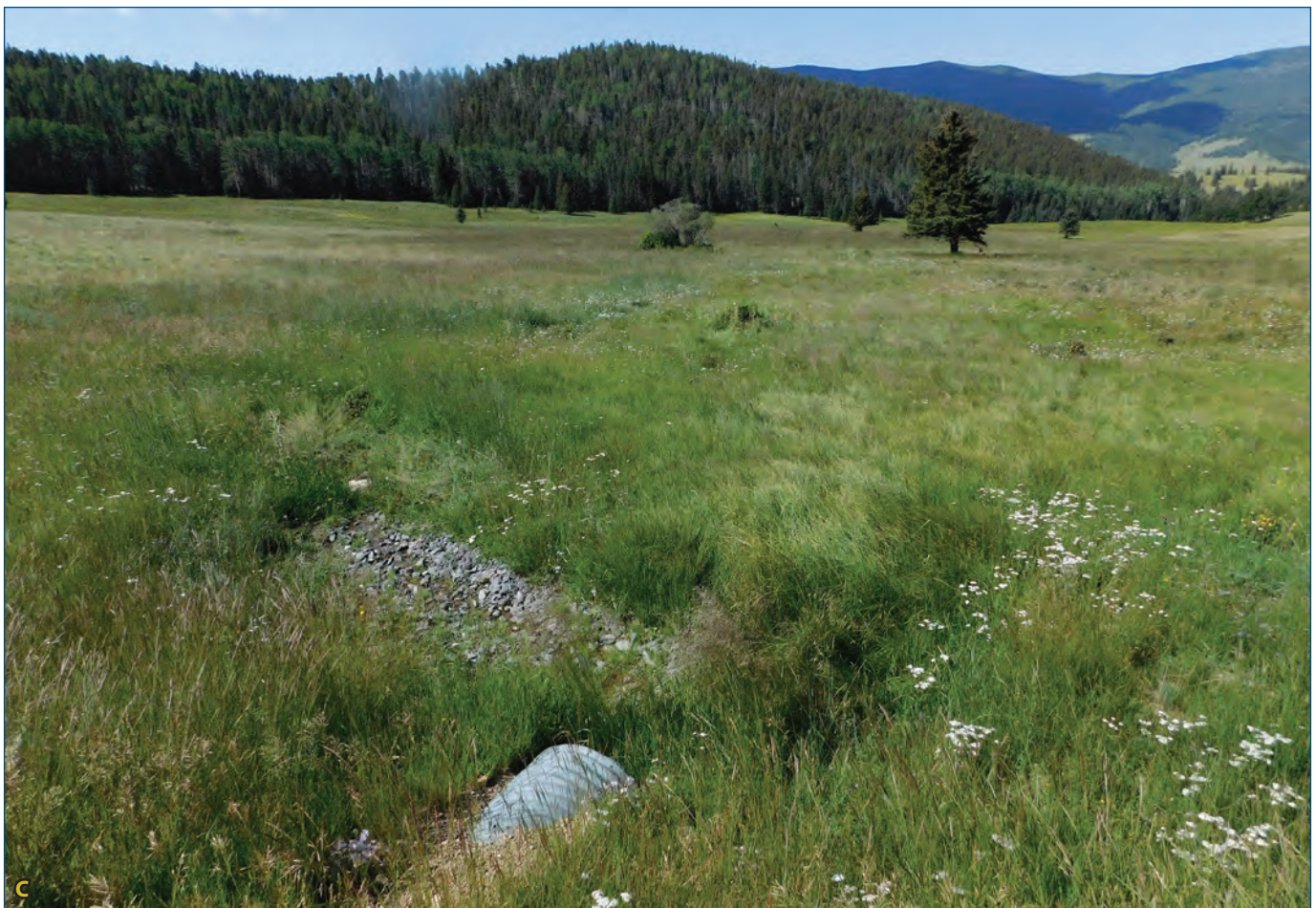
Figure 4.20A. This photo shows sediment deposition from a culvert constricted flow path over an alluvial fan. Figure 4.20B. The sediment deposit was removed and a reinforced spreader swale was installed to convert concentrated outflow from the culvert into sheetflow over a greater area. Blue arrows indicate flow paths. Figure 4.20C. After one good water year, the restored sheetflow into the wider area resulted in more productive vegetation.
