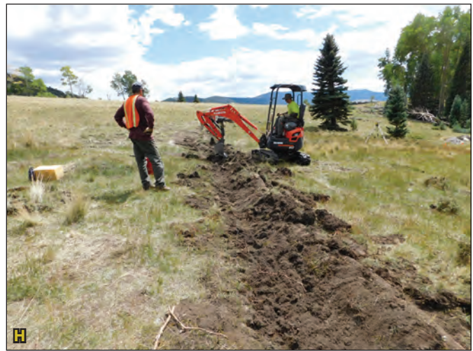
Figure 4.10G. Elevations were surveyed so that the swale was not at too steep an angle on the hillslope, which would have caused erosion. This also created a swale that followed the natural topography and not a straight line across the slope. Blue arrows indicate flow paths. Figure 4.10H. The logs were keyed into the soil surface to minimize piping (leakage) underneath, then covered with sod.
