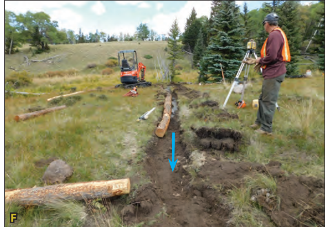
Figure 4.10E. A rock reinforced berm keeps the water in the swale. Figure 4.10F. Logs were buried in the downvalley edge of the swale to create a slightly higher berm. Blue arrows indicates flow paths.
