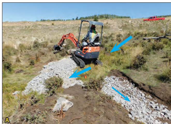
Figure 4.19A. A rock flow splitter was constructed in this incised channel to direct water concentrated by an up-gradient culvert into an abandoned stock pond. Blue arrows indicate flow paths. Figure 4.19B. Adaptive management was implemented with larger rocks to raise the elevation of the flow splitter the year after the splitter was installed, so that it could perform as intended.
