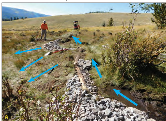
Figure 4.11A. The constructed keypoint diverts water from the channelized source via a lead-out berm to a reinforced spreader swale, sheetflow spreading structure, and stable return. Figure 4.11B. This photo shows sheetflow below a stable return. Blue arrows indicate flow paths.
