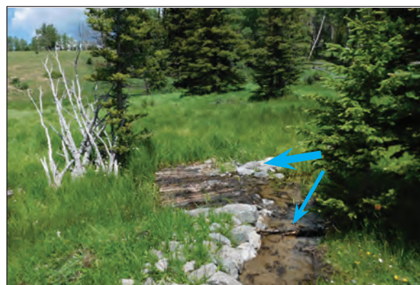
Figure 4.1. A log step fall to stabilize a headcut is elevated to split channel flow to a lead-out berm. The lead-out berm was excavated a few inches deep to achieve a suitable elevation for capturing and directing the flow that was split from the main channel. Blue arrows indicate flow paths.
