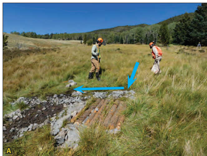
Figure 4.15A. In East Holman Creek, an incised channel with high and dry banks was mechanically collapsed to form a modified channel, which was armored with cobbles and integrated with down-gradient stabilization and flow-spreading structures. Figure 4.15B. In June of the following year, the structure was functioning properly to spread sheetflow to the former wetland on valley right. Blue arrows indicate flow directions.
