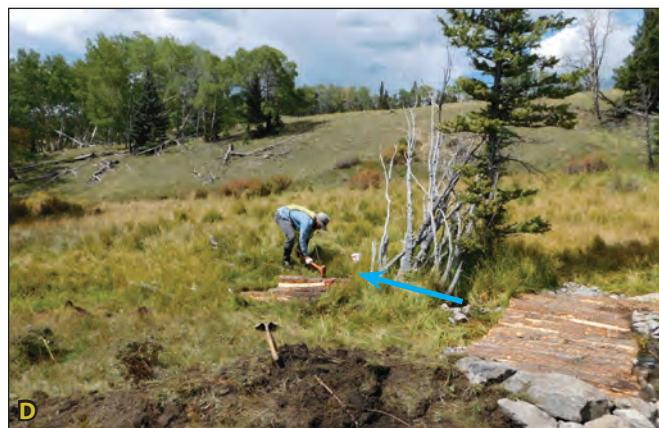
Figure 4.10A. The location for the log mat flow splitter was surveyed to ensure that water could be moved out of the channel at the proper elevation. Figure 4.10B. A swale was created to receive the water diverted from the channel by the log mat flow splitter. Figure 4.10C. The log structure diverts water to the swale. Figure 4.10D. A log mat is installed in the main channel below the flow splitter to raise the grade of the incised channel and further spread water over the wetland surface. Blue arrows indicate flow paths.
