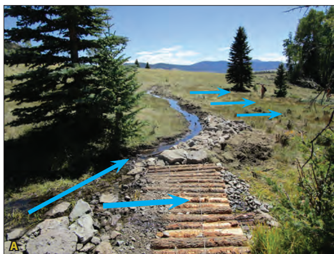
Figure 4.7A. A log step fall in West Holman Creek, serving as a flow splitter, stabilizes a head cut and splits water flow into an armored lead-out channel to a reinforced spreader swale, while allowing some flow to remain in the current channel to support downstream wetland vegetation. The log step fall is the constructed keypoint. Figure 4.7B. After one year, the swale is allowing water to both infiltrate below the berm and spill past a stable return at the end of the berm to rewet former wetland. Figure 4.7C. In this photo, sheetflow from the upstream lead-out swale and berm (Fig. 4.7A) is visibly travelling downvalley past the large and seedling conifers visible in these pictures (white arrows). Blue arrows indicate flow paths.
