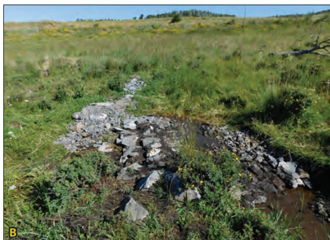
Figure 4.19A. A rock flow splitter was constructed in this incised channel to direct water concentrated by an up-gradient culvert into an abandoned stock pond. Blue arrows indicate flow paths. Figure 4.19B. Adaptive management was implemented with larger rocks to raise the elevation of the flow splitter the year after the splitter was installed, so that it could perform as intended.
