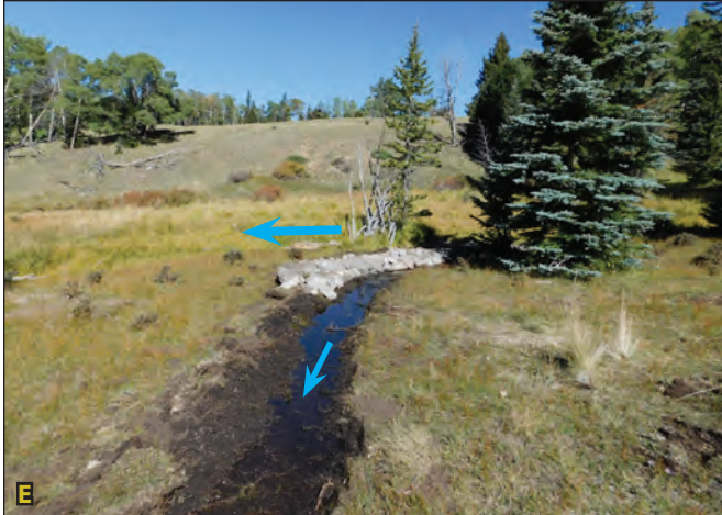
Figure 4.10E. A rock reinforced berm keeps the water in the swale. Figure 4.10F. Logs were buried in the downvalley edge of the swale to create a slightly higher berm. Blue arrows indicates flow paths.
