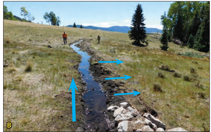
Figure 3.14A. The presence of Juncus (brownish-green colored rush) in the otherwise upland vegetation indicated that it might be possible to return this area to wetland obligate vegetation with increased water infiltration to the soil. Figure 3.14B. The photograph shows a constructed swale and berm at the end of a lead-out berm which moves water to the farthest extent possible. The treatment will increase water infiltration downvalley. Blue arrows indicate flow paths.
