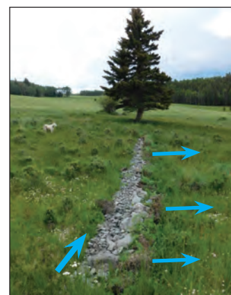
Figure 4.6. This swale was lined with angular cobble to increase stability because the wet meadow vegetation is currently not adequate to hold soil in a large flow event. Additional armoring is necessary until the swale has had some time to spread water and convert the dessicated wet meadow to wetland vegetation. Armoring also provides much needed protection from animal impacts, especially hoof shear. Blue arrows indicate flow paths.
