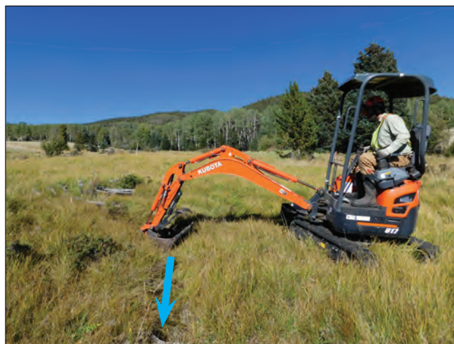
Figure 4.13. An incised channel bisecting this slope wetland complex in East Holman Creek has lowered the localized water table and caused the bank vegetation to dry out, leaving the channel vulnerable to further degradation. The channel is being stabilized by using a mini-excavator to collapse the high banks in order to raise the grade. Blue arrow indicates flow direction.
