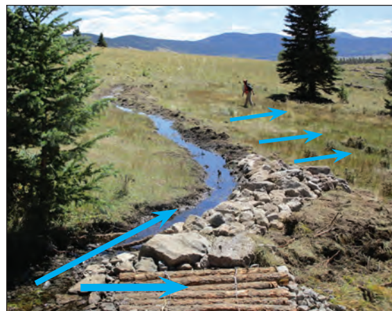
Figure 4.9. A rock armored lead-out berm and excavated channel split flows into a log reinforced spreader swale in the West Holman Creek drainage. Blue arrows indicate flow paths.
