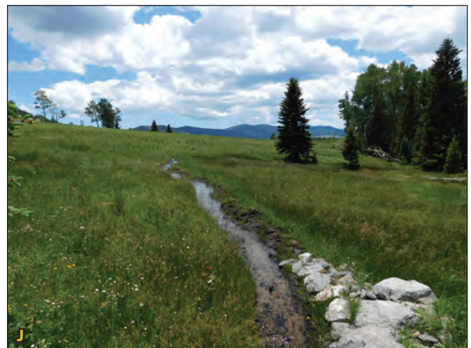
Figure 4.10I. One day after completion of the treatment train, water reaches the far end of the swale and berm structures. Figure 4.10J. After one year, the structures are saturating the former wetland downslope.
