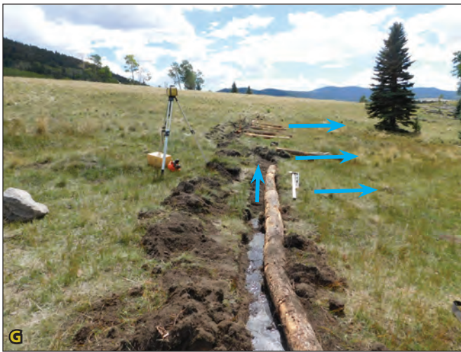
Figure 4.10G. Elevations were surveyed so that the swale was not at too steep an angle on the hillslope, which would have caused erosion. This also created a swale that followed the natural topography and not a straight line across the slope. Blue arrows indicate flow paths. Figure 4.10H. The logs were keyed into the soil surface to minimize piping (leakage) underneath, then covered with sod.
