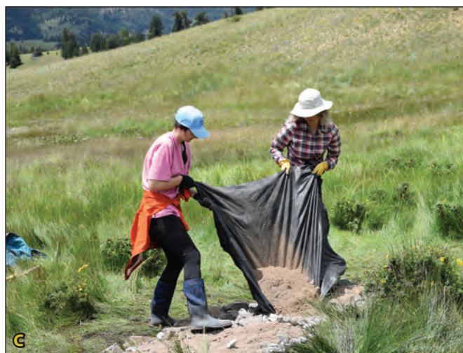
Figure 4.5A. The photo above shows Carex growing through a log mat. Figure 4.5B. These structures had base course materials used to key them together. Base course remains on the wetland surface. Blue arrows indicate flow directions. Figure 4.5C. shows Geotextile fabric being used to deliver finer materials to stabilize a media luna with no impact to the surrounding wetland vegetation.
