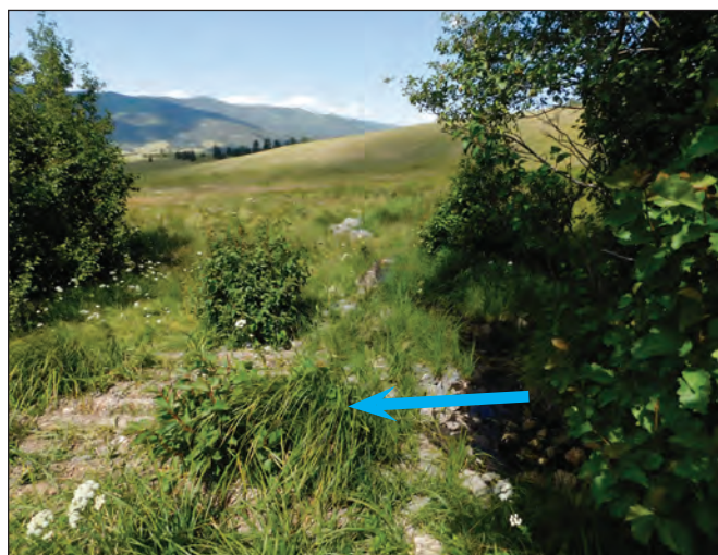
Figure 4.3. This log mat flow splitter was built upstream of a large headcut. It spreads the majority of flow to valley right through a rock and log reinforced lead-out berm. Existing vegetation was carefully incorporated into the flow splitting structure and new vegetation is colonizing the treatment area. The downstream area is kept saturated but the flow splitter prevents it from receiving erosive flows. Blue arrow indicates flow direction.
