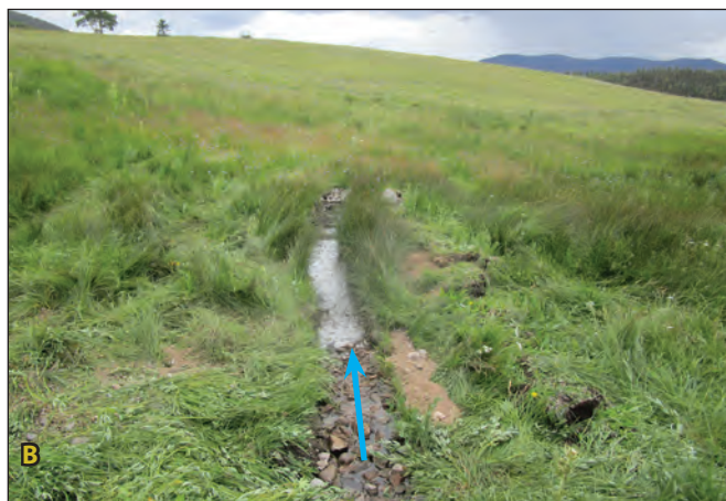
Figure 4.16A. This photo shows a non-functioning stock pond with a breached berm (yellow line) in Middle Holman Creek. Figure 4.16B. This photos shows the breach plugged. A treatment train was installed at the pond spillway to send water to drying wetlands on valley right. Blue arrows indicate flow directions.
