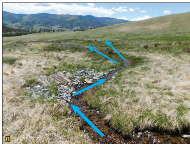
Figure 4.15A. In East Holman Creek, an incised channel with high and dry banks was mechanically collapsed to form a modified channel, which was armored with cobbles and integrated with down-gradient stabilization and flow-spreading structures. Figure 4.15B. In June of the following year, the structure was functioning properly to spread sheetflow to the former wetland on valley right. Blue arrows indicate flow directions.
