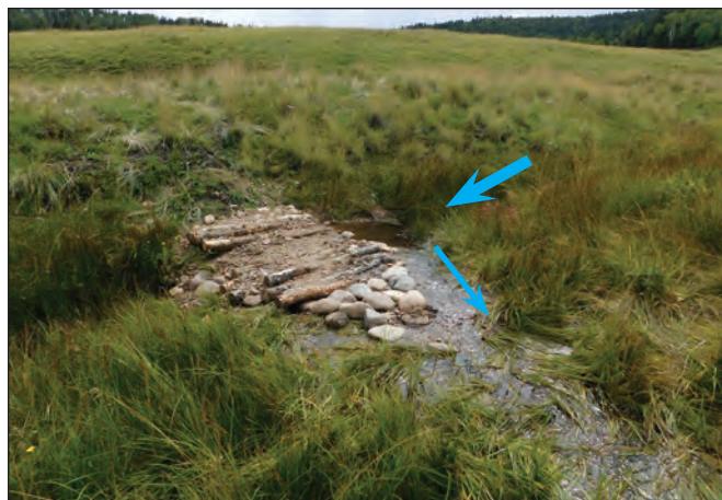
Figure 4.2. This log and rock flow splitter is built higher on the upstream side to spill water out of the incised channel and back onto the wetland surface. Blue arrows indicate flow paths.
