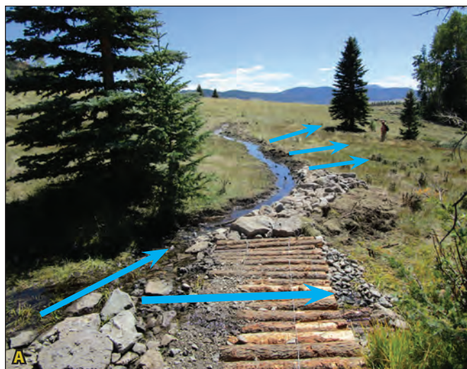
Figure 3.10A. This example of a treatment train begins with a log mat flow splitter connected to a rock armored lead-out berm moving water into a swale with a log and sod reinforced berm. Figure 3.10B. The treatment train culminates in a stable return composed of two rock media lunas that spread water across the target area. Blue arrows indicate flow directions.
