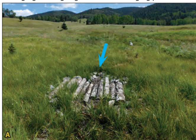
Figure 4.5A. The photo above shows Carex growing through a log mat. Figure 4.5B. These structures had base course materials used to key them together. Base course remains on the wetland surface. Blue arrows indicate flow directions. Figure 4.5C. shows Geotextile fabric being used to deliver finer materials to stabilize a media luna with no impact to the surrounding wetland vegetation.
