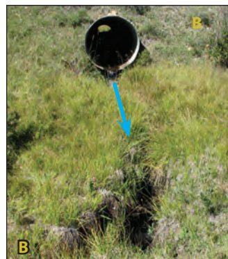
Figure 3.9A. Aerial image of East Holman Creek bisected by Forest Service Road 1950. Figure 3.9B. A culvert concentrates flow, causing the channel to downcut below the culvert. Blue arrow indicates flow path. Figure 3.9C. An old stock pond interrupts sheetflow through the hillslope. Yellow line indicates approximate top of pond berm.
