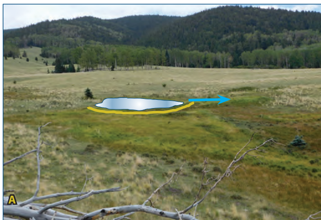
Figure 4.16A. This photo shows a non-functioning stock pond with a breached berm (yellow line) in Middle Holman Creek. Figure 4.16B. This photos shows the breach plugged. A treatment train was installed at the pond spillway to send water to drying wetlands on valley right. Blue arrows indicate flow directions.
