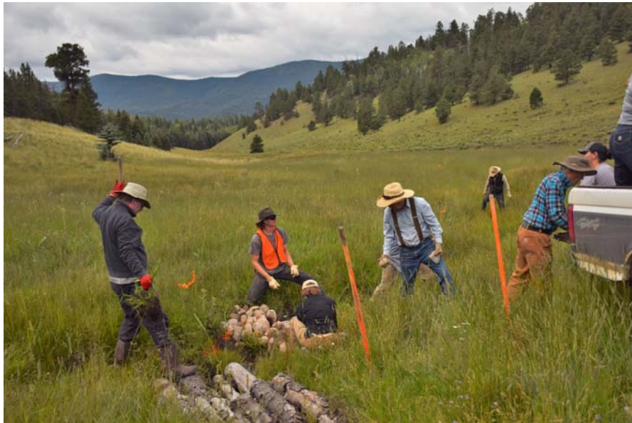
Quivira Coalition building one-rock dams to capture sediment and raise water table in slope wetlands in the Comanche Creek Watershed
