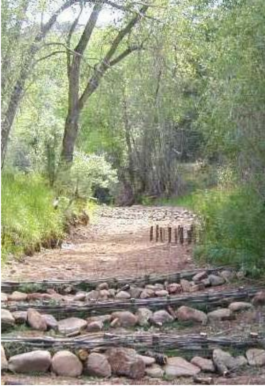
Figure 24. “Pole baffle” (back) and “wicker weirs” (front) installed to capture sediment and recreate riffle/pool sequence and meanders in Galisteo Creek.
