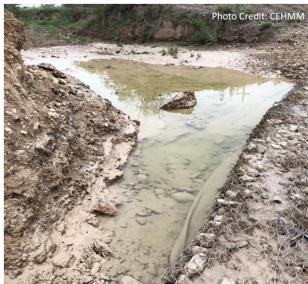
Figure 42. A blow out on the banks of the Black River after a larger rain.
