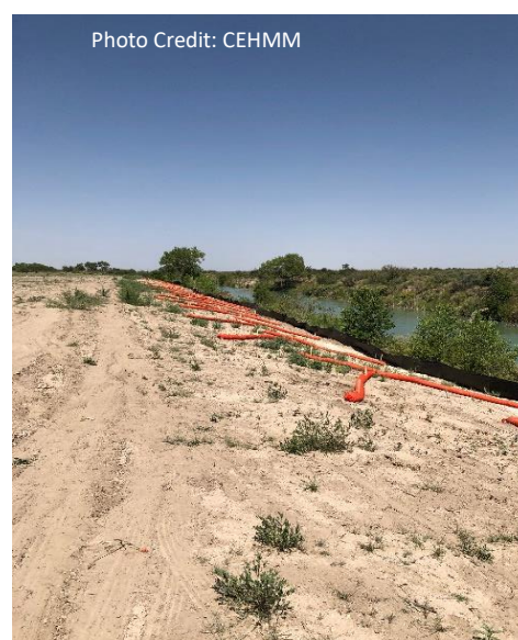
Figure 37. Completed erosion mitigation project on the Black River with silt fence and filter socks installed.
